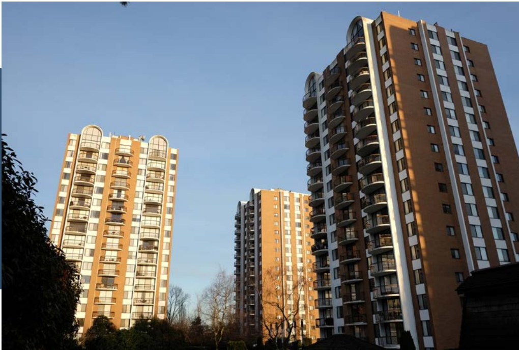
Existing towers at Langara Gardens
