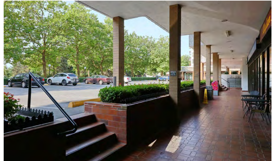
Langara Gardens, existing retail condition
