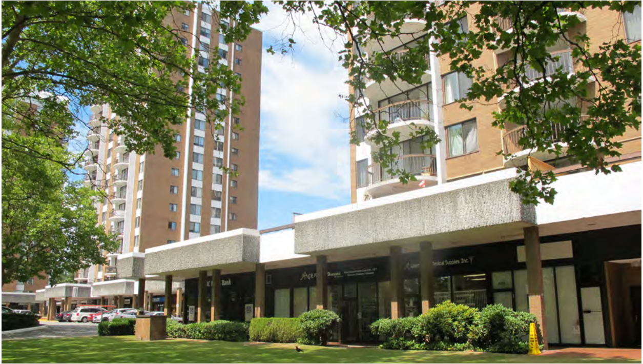
Retail podium along West 57th Avenue
