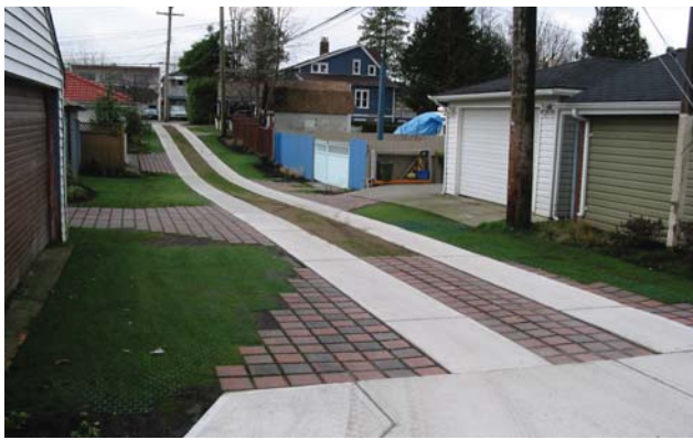
Laneway designed with natural stormwater management features.
