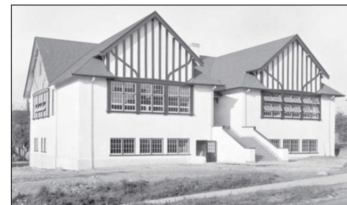
123 E 6th Avenue (City-Owned) Simon Fraser Annex Built 1929
