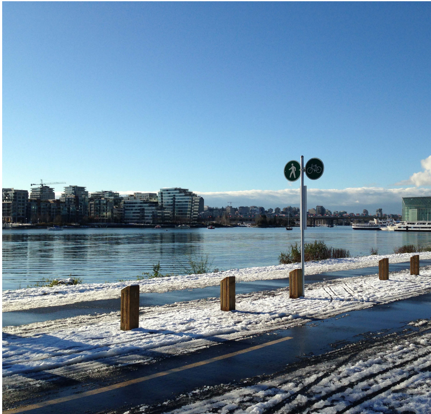
Existing Seawall at NEFC site.
