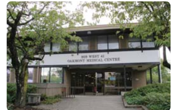
Oakmont Medical Centre
