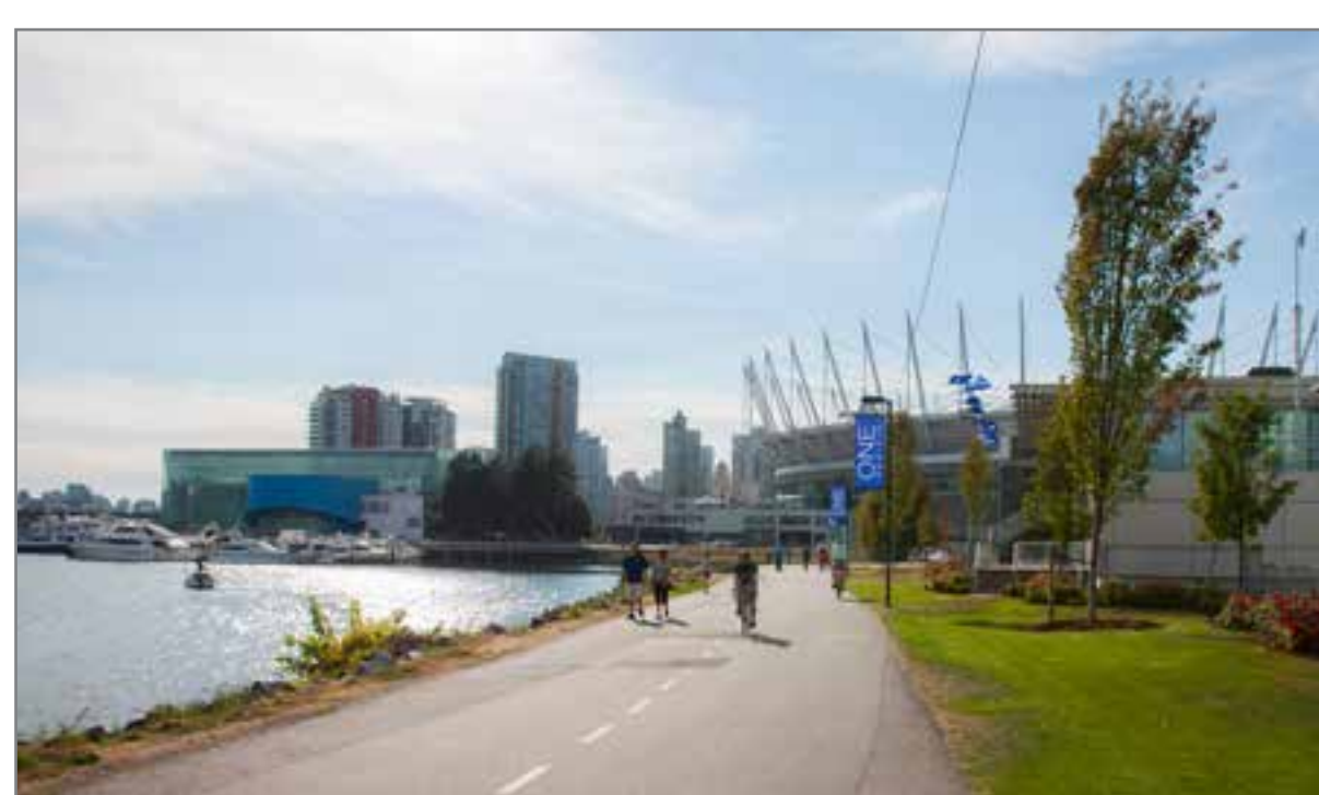
Interim Seawall Improvements
