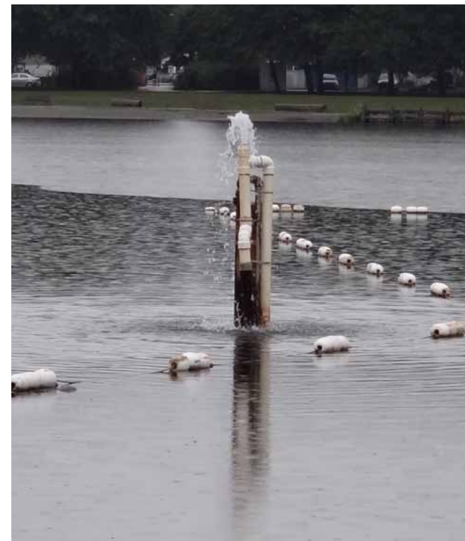
It is recommended that the existing potable water input be replaced.
