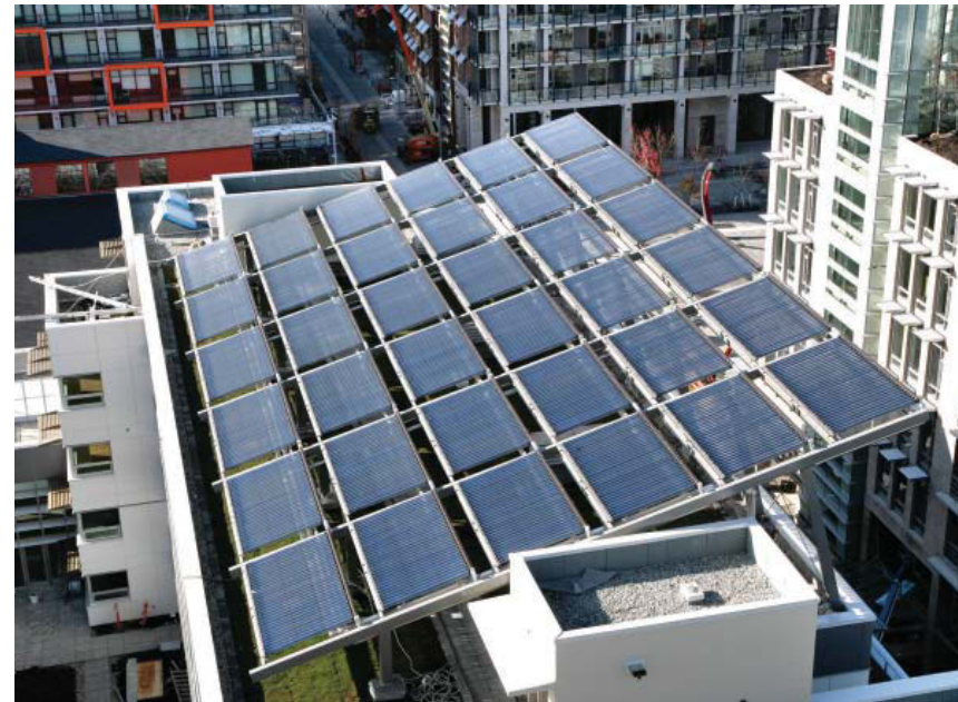
Solar collector on roof of affordable housing building
