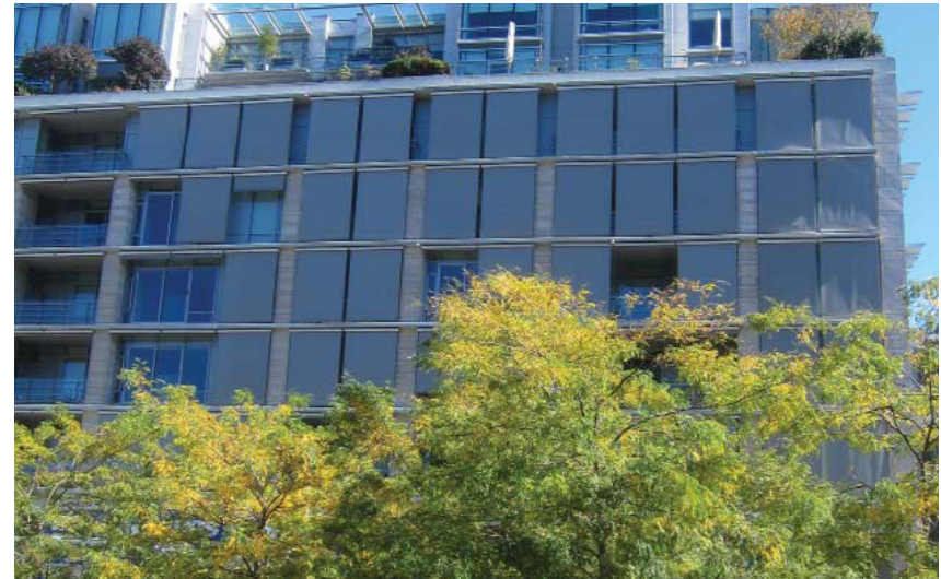
Building with solar shading
