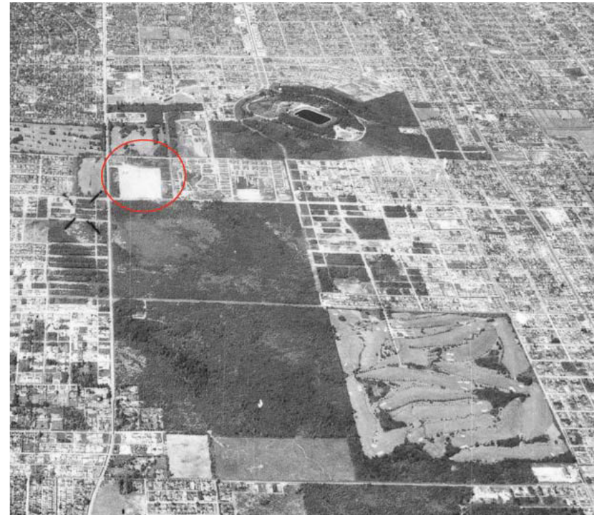
Aerial photograph showing the context of the OTC (June 1948)
