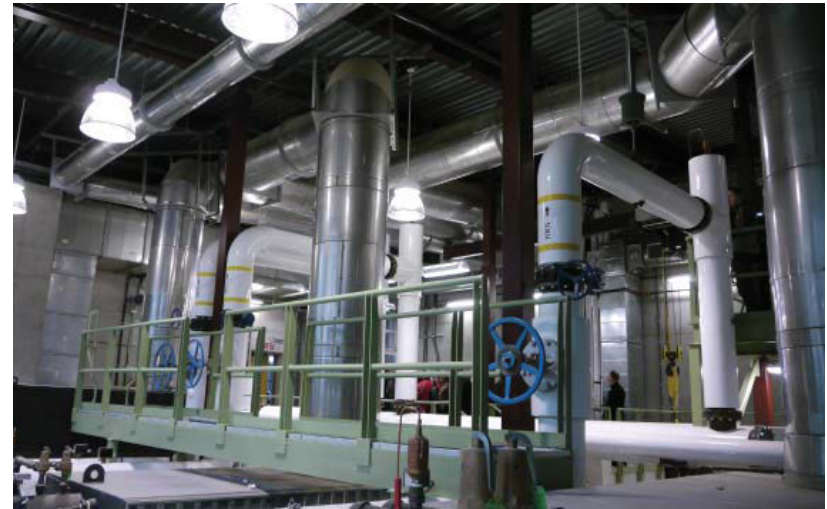
Neighbourhood energy utility
