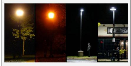
The image above illustrates four different outdoor light fixtures with a person standing beneath each one. The subject is much more visible in the two images on the right, which show *full cut-off* fixtures.
