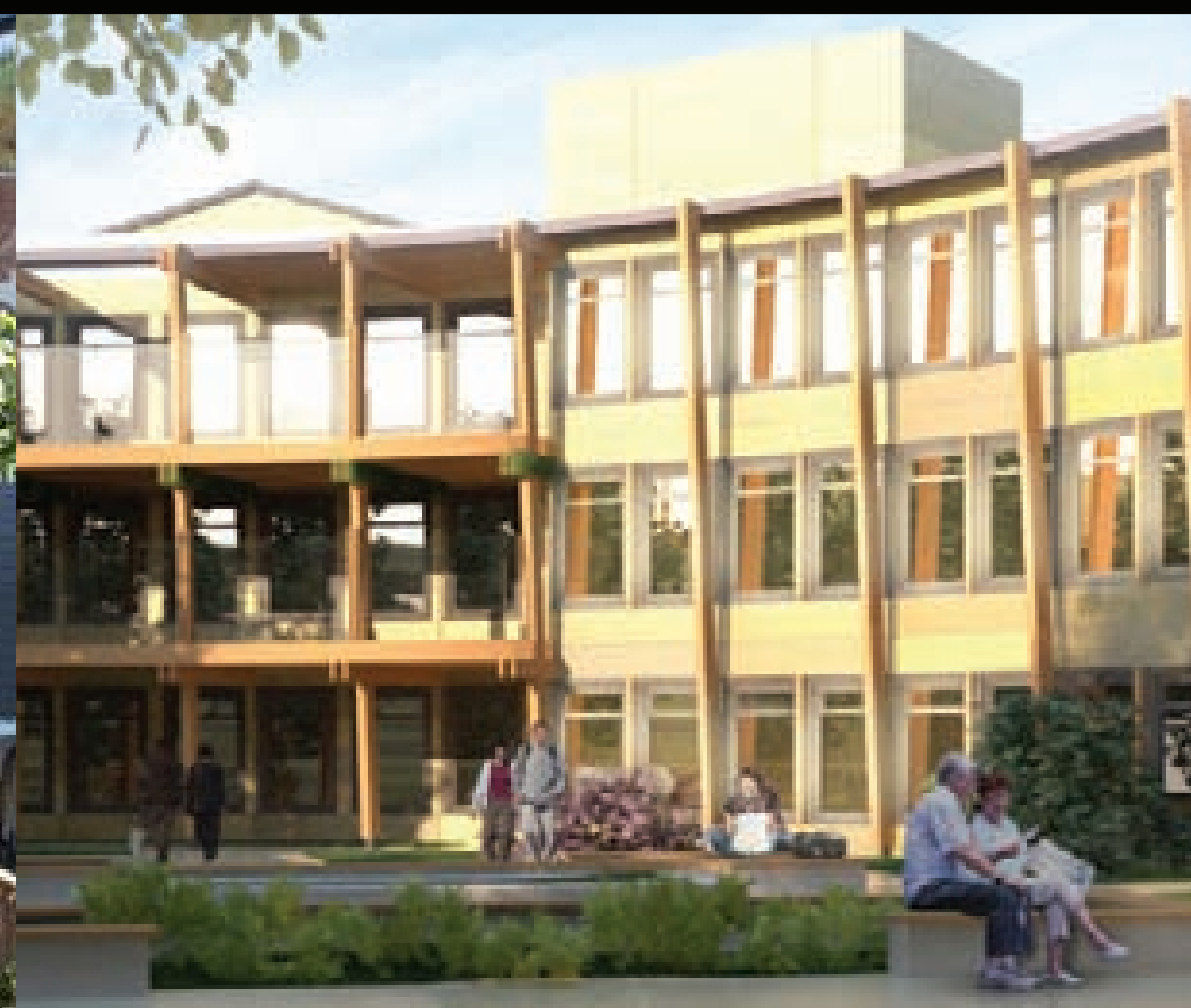
Complex Residential Care
