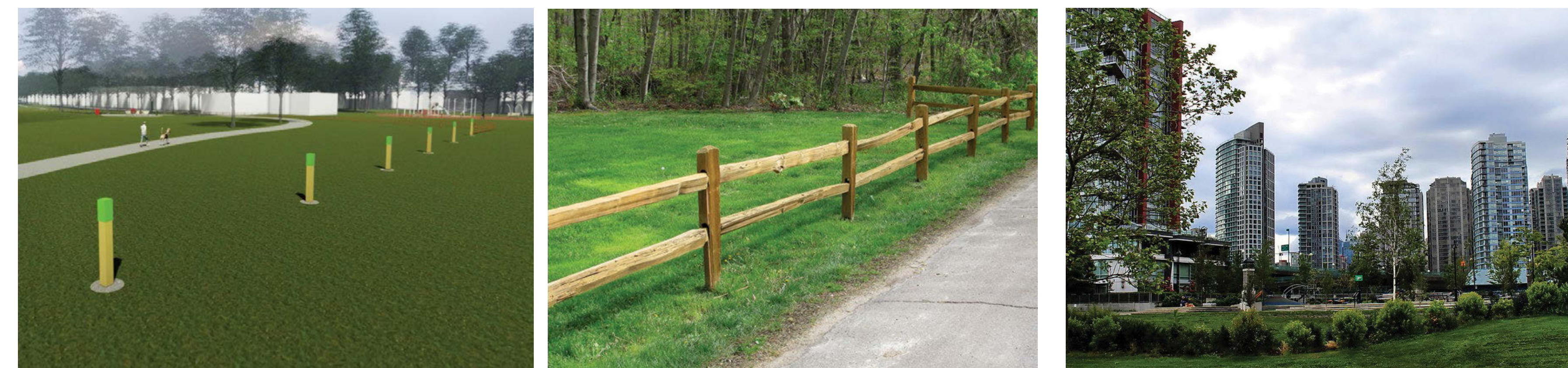
Non-secure boundaries: bollards, in wood or steel (left), post and rail fencing (center), or vegetation (right) where secure containment is not required.
