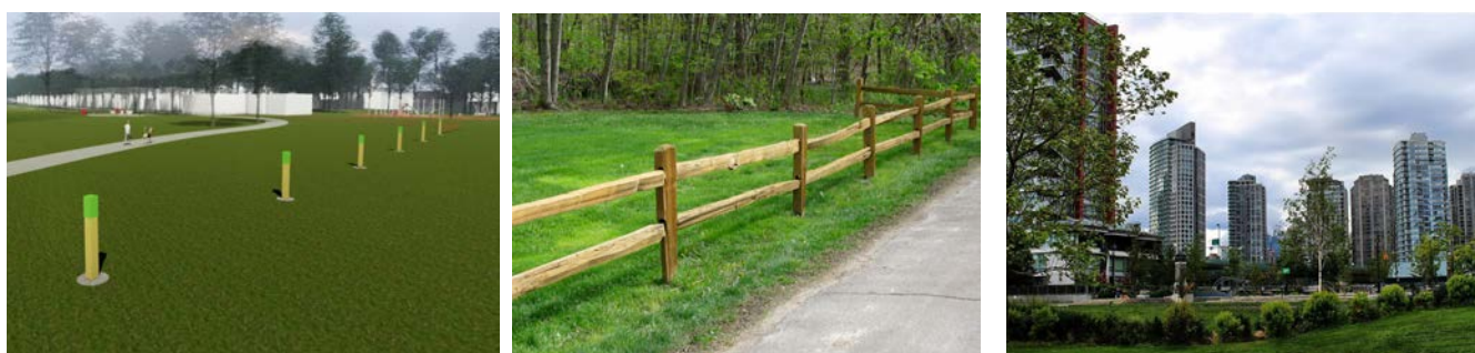
Non-secure boundaries: Bollards, in wood or steel (left), Post and rail fencing (centre), or vegetation (right) where secure containment is not required
