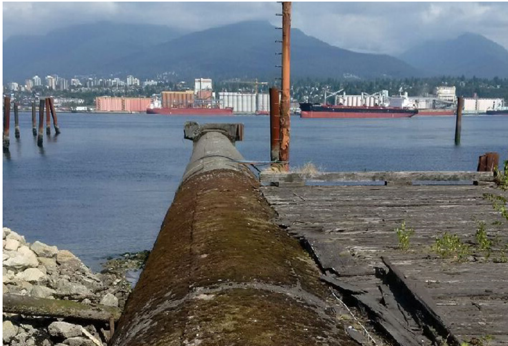
Removing rainwater from sewer pipes will reduce combined sewer overflows. City must eliminate CSOs by 2050.
