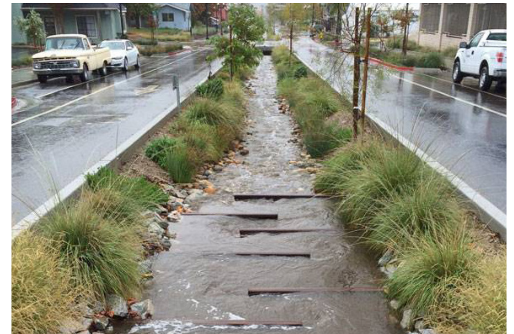
21st Street, California. Integrated bioswale.
