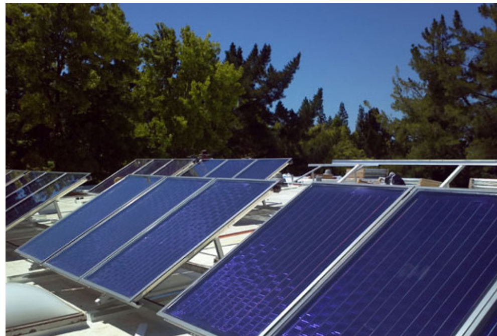
Solar panels are a common renewable energy solution that has been integrated with buildings for many years.
