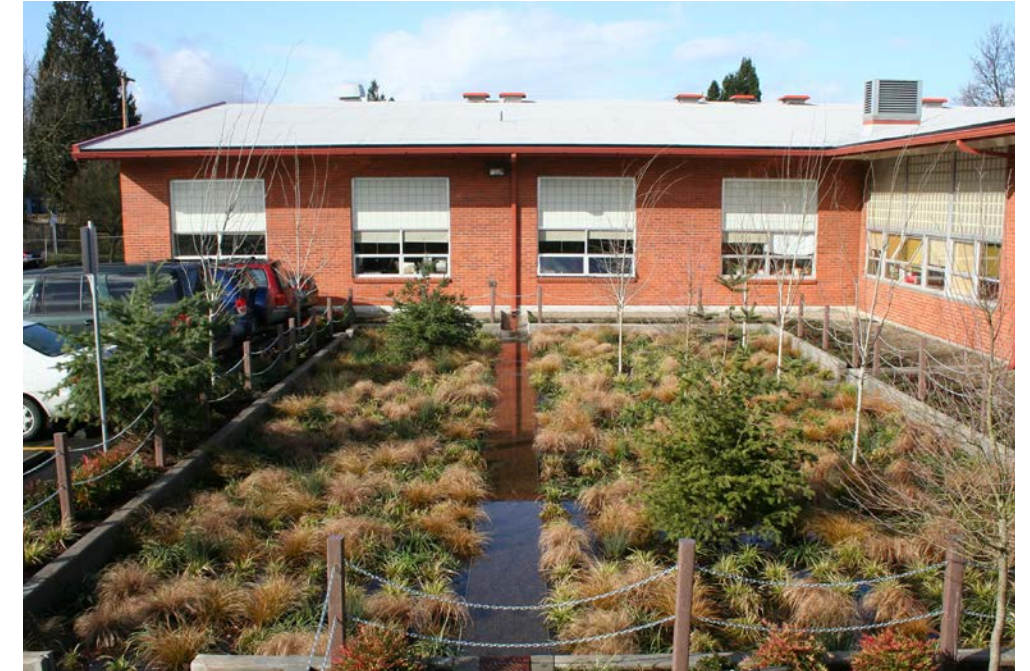
Mount Tabor Middle School, Oregon. Rain Garden that reduces rainwater surface run-off.
