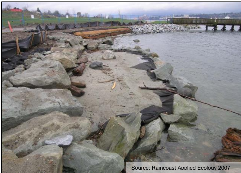
Photo 2 Completed Shoreline Stabilization with Dune Grass Bench in Foreground Bioengineered and Boulder Banks in Background (facing west)
