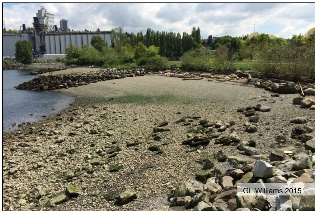
Photo 4 Rock Groynes Separating Scalloped Intertidal Beaches with Varying Substrates and Boulder Banks Looking East
