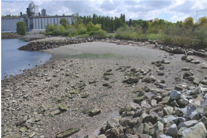
Photo 1. Extended rounded rock groins separating scalloped intertidal beaches.
