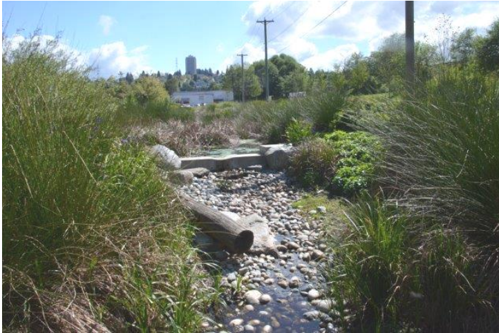
Photo 13. Daylighted Renfrew Creek showing weir and cobble-gravel lined channel in Creekside Park.
