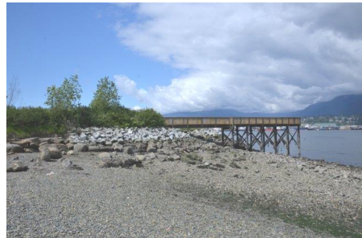
Photo 4. Timber pile supported observation deck at the western limit of study area.
