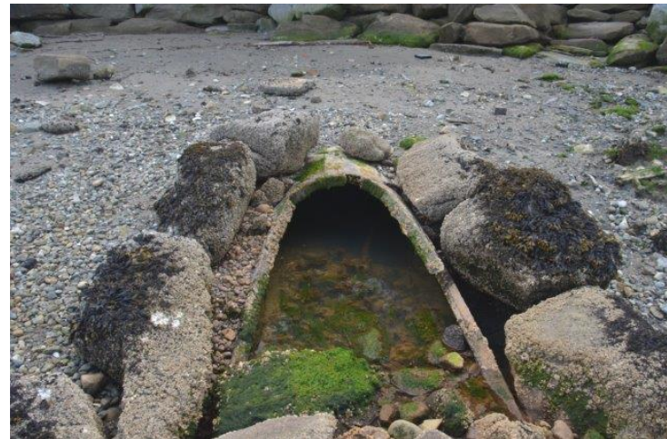
Photo 16. Wooden culvert beach outlet of Renfrew Creek that discharges into Burrard Inlet.
