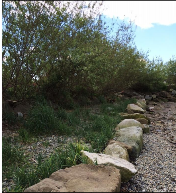
Photo 5 Dune grass Bench Created with Boulders and Sand Fill below Riparian Shrub Backshore Habitat
