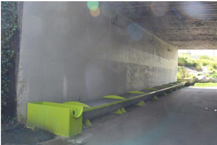
Photo 15. Aboveground flume transports flows from daylighted stream to underground culvert that discharges into Burrard Inlet.
