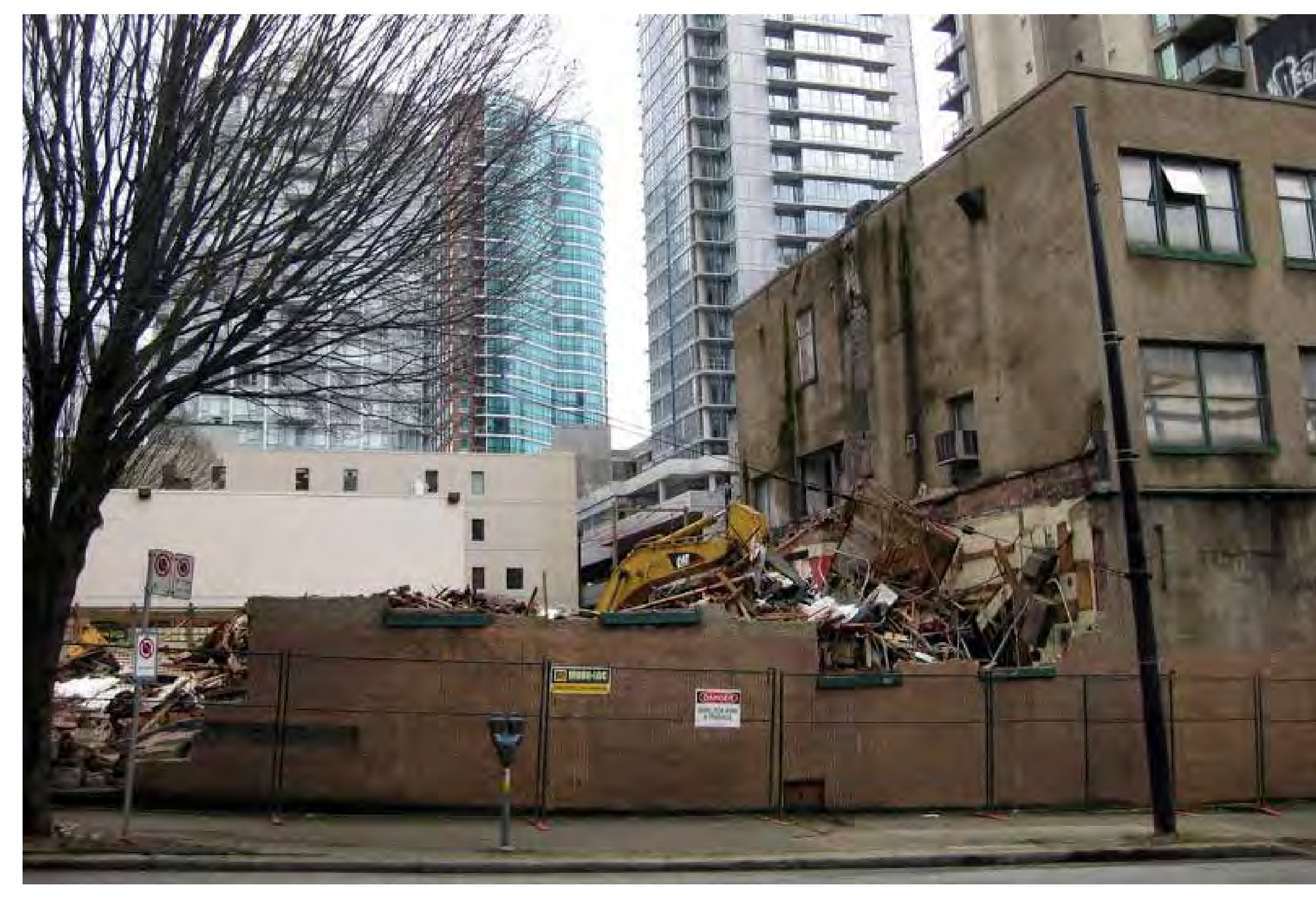
Demolition of the building at the south part of the site at Smithe Street (early 2000s)
