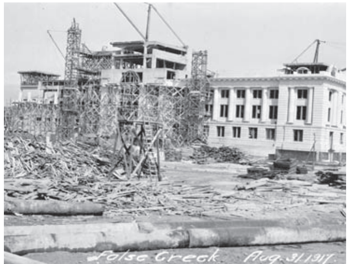
Constructing the CNoR Terminal, August 1917, CVA BuN540.051
