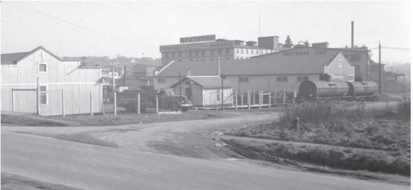
Restmore Manufacturing Building, 1000 Parker Street, ca. 1940s, CVA 1184-1699
