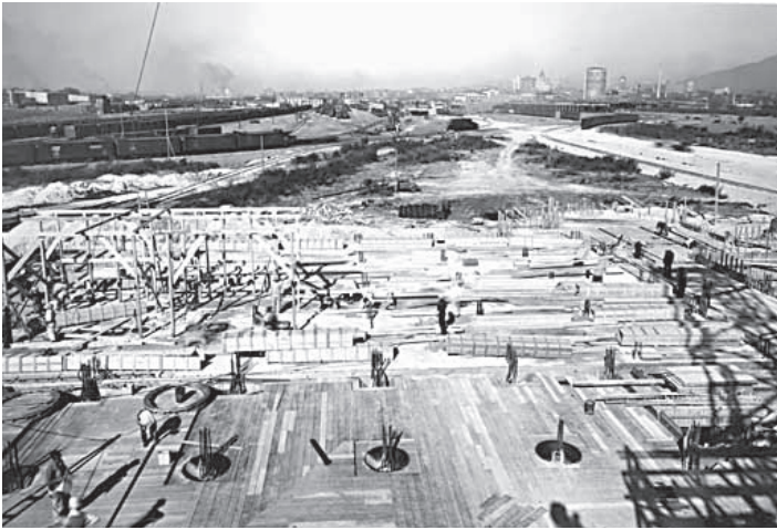
Canada Packers under construction, September 1937, VPL 12239
