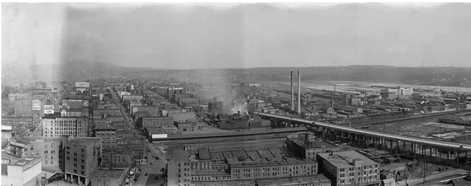
Original Georgia Street Viaduct, ca. 1921, CVA PAN N221
