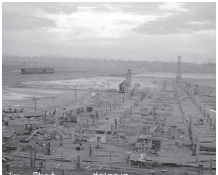
Rail Shed Construction on the False Creek Flats, March 1917, CVA A09081
