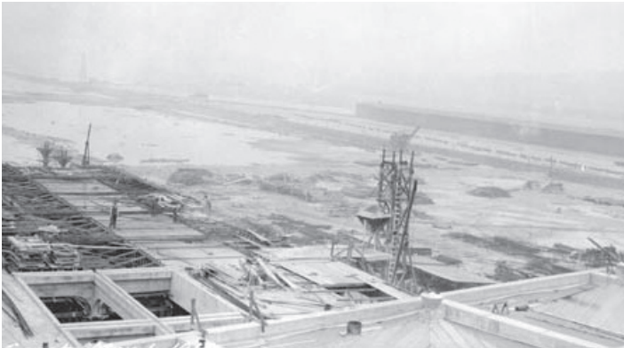
Filling the flats and constructing the CNoR Terminal, 1918, CVA Bu N540.094
