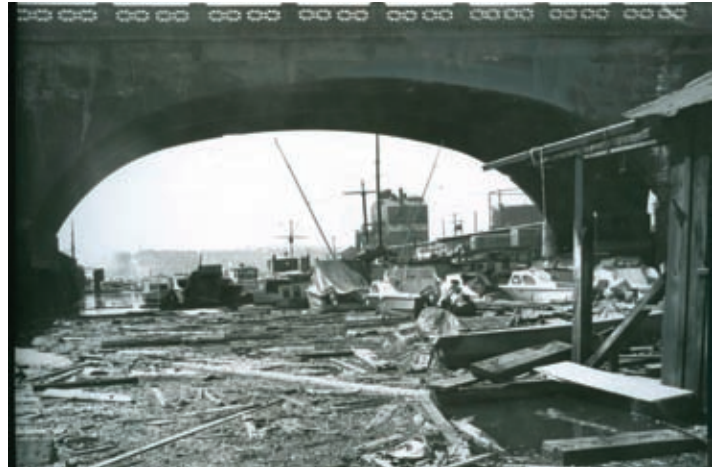
Debris beneath the original Georgia Street Viaduct, 1961, Vancouver Sun
