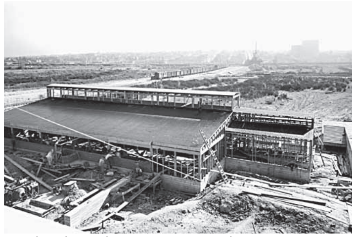
Canada Packers under construction, September 1937, VPL 12240
