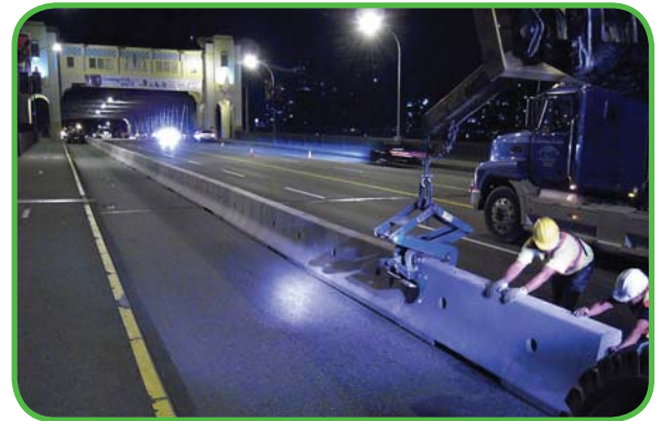
Temporary protective barriers were installed to separate cycling and vehicle lanes.
