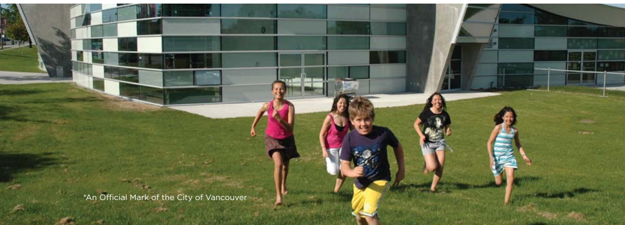
SUNSET COMMUNITY CENTRE Varied glass panels control sunlight and heat entering the building.
