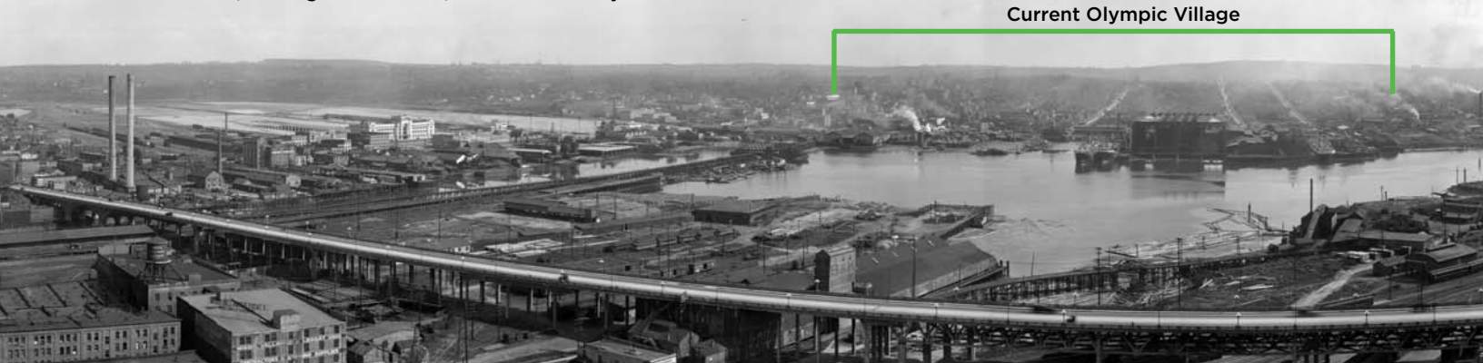
False Creek, looking south in 1921, W.J. Moore - City Archives
