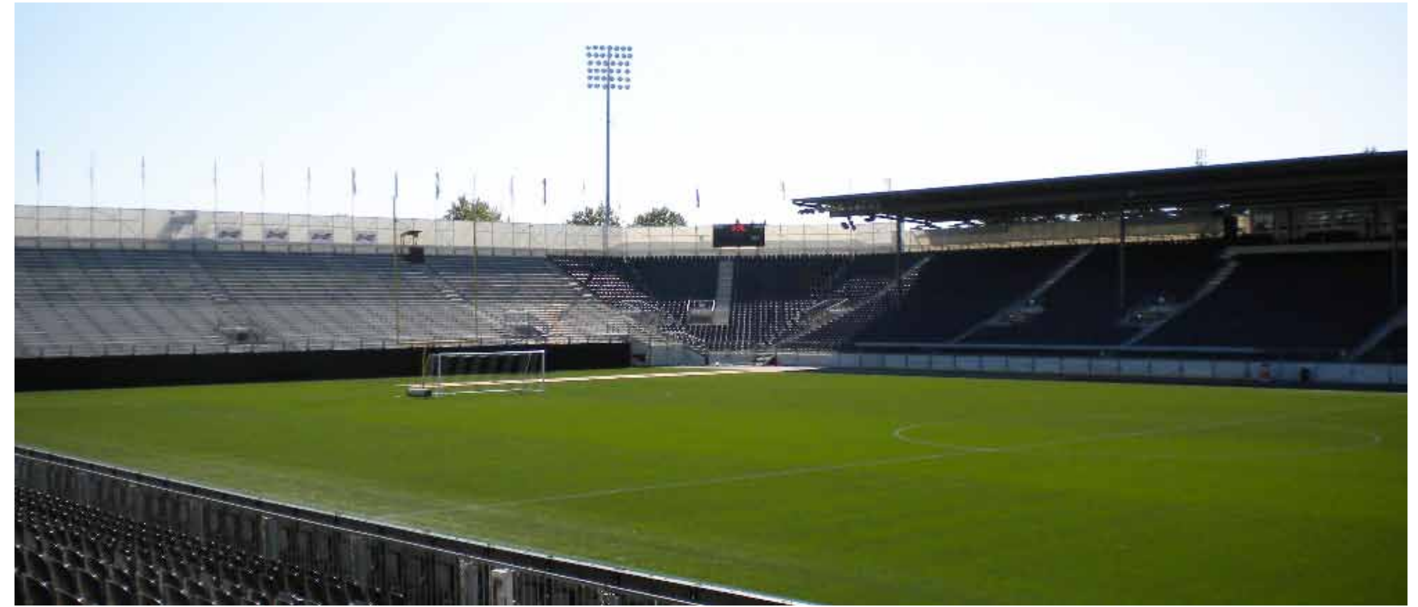
Temporary Stadium and High Mast Lights
