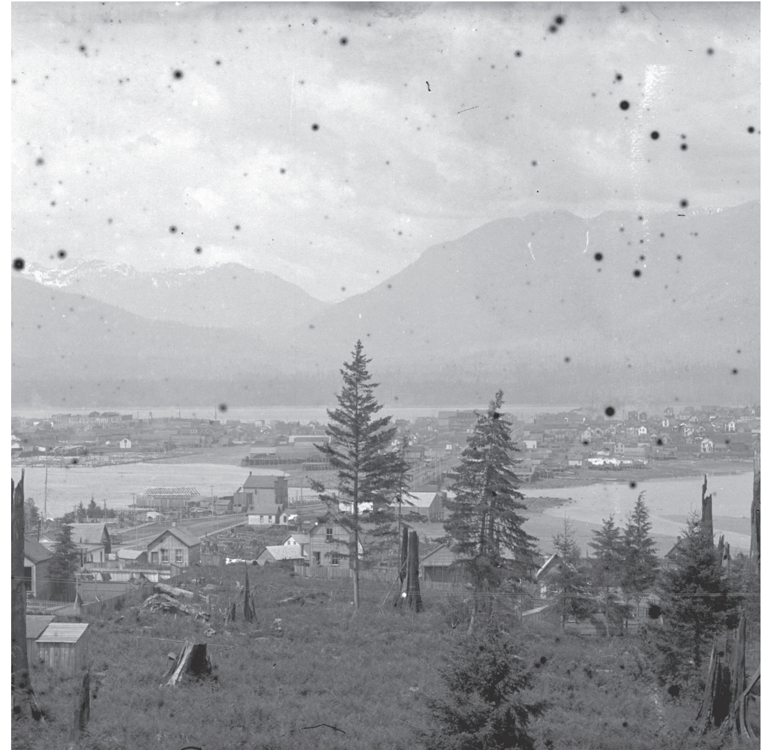
Looking north from Mount Pleasant at False Creek. Westminister Bridge (now Main Street) circa 1890s. City of Vancouver Archives
