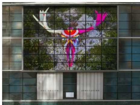
4. Dal Grauer Substation al'taqiaq, Jordan Bennett, 2020
