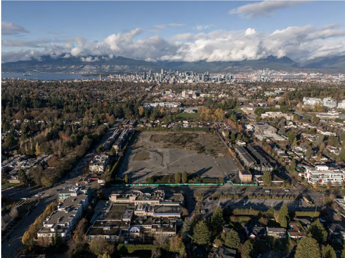
Figure 01 Looking due north with West 41st Avenue in the foreground and the OTC site in the fore- and mid-ground, downtown Vancouver in the background
