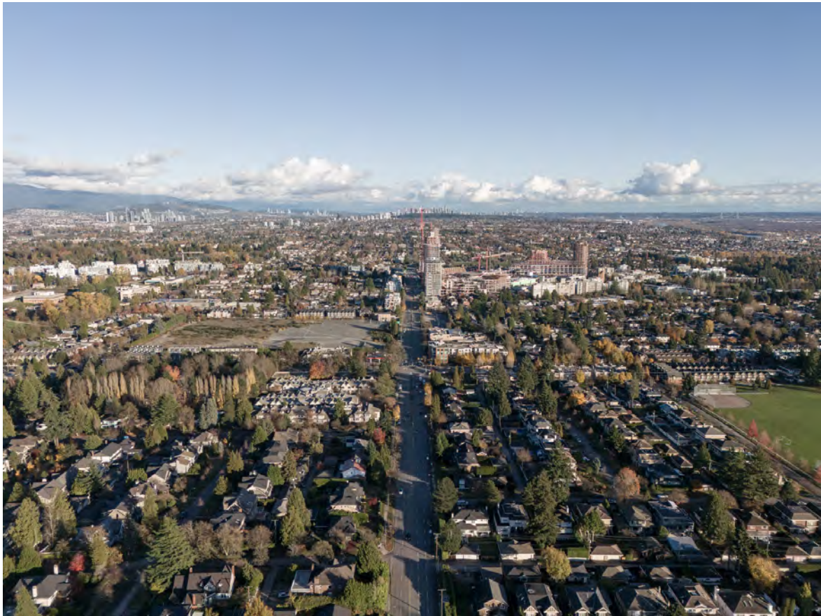
Figure 38 Looking due east down West 41st Avenue with the OTC site in the mid-ground and Metrotown Town Centre in Burnaby in the background
