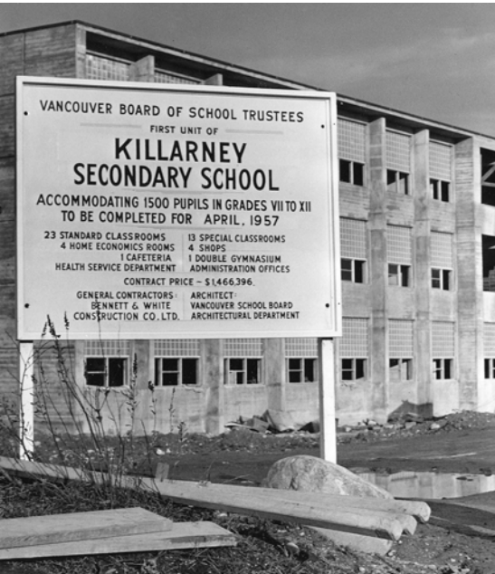
Killarney Secondary School Site, 1950's
