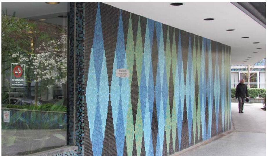
BC Binnings, BC Hydro Building, Vancouver BC
