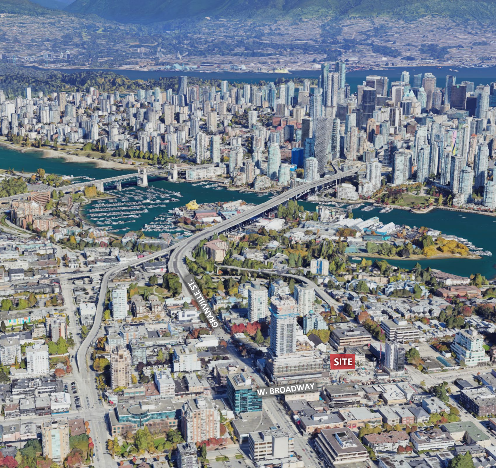
Aerial view of development site
