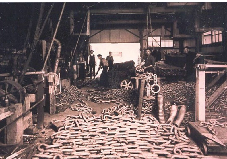
Canada Chain and Forge Company on Granville Island, c.1929
