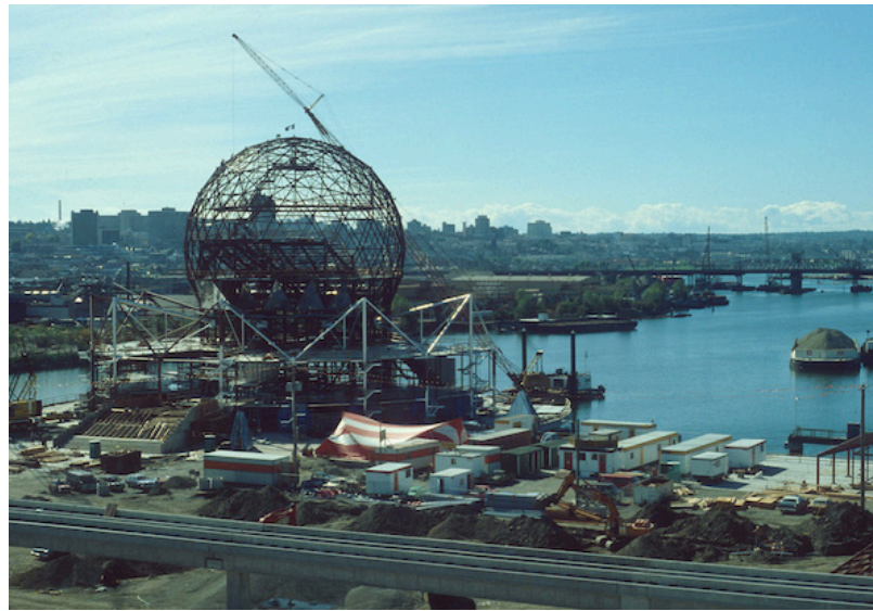
Science World geodesic dome in construction, 1984
