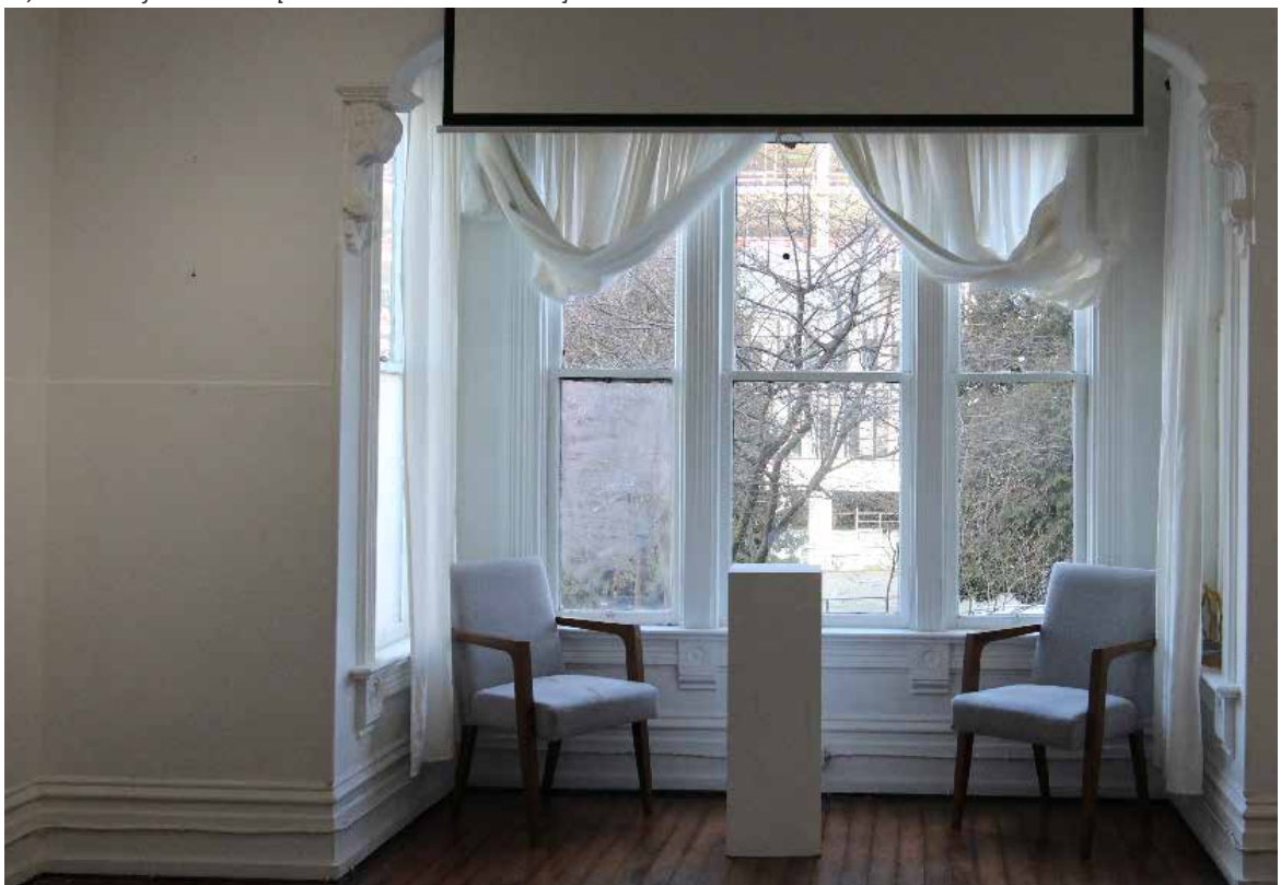
Arched opening to bay window with ornamental plaster corbels and baseboards, as viewed from interior [Donald Luxton & Associates]
