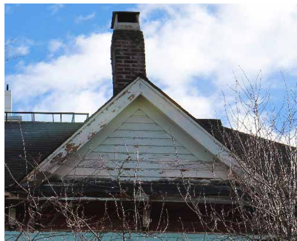
Close-up of noted narrow wood dropped siding [Donald Luxton & Associates]
