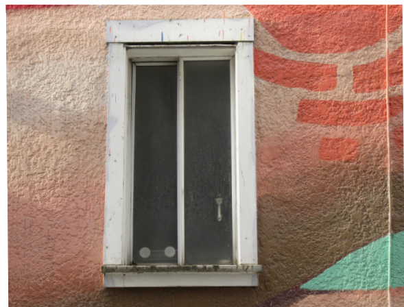
Existing window opening on east elevation, insert window installed.
