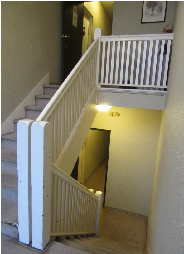
Open wood balustrade with square spindles and wood newel post.
