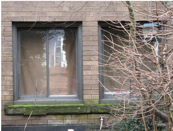
Original double assembly window openings on basement level with sandstone sill.
