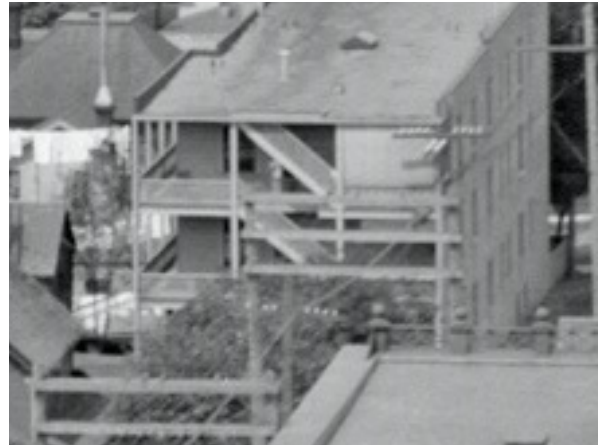
1913. Moore, W.J. Panorama of Vancouver [CVA PAN N161A] showing Donnacona Block's original wraparound balconies, exterior stairs and roof overhang. Rear exit doors are hidden by stairs.
