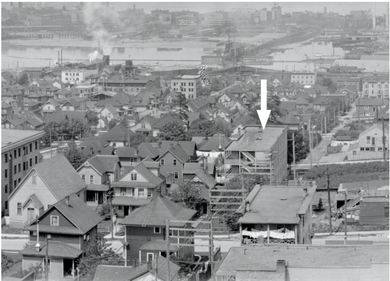
1913. Moore, W.J. Panorama of Vancouver [CVA PAN N161A]. Connaught Bridge, later known as Cambie Street Bridge. Mount Pleasant shown in foreground and downtown Vancouver beyond. Donnacona Block shown by white arrow.
