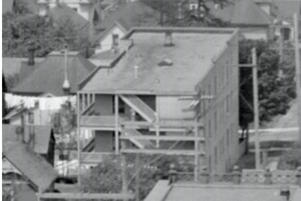
1913. Moore, W.J. Panorama of Vancouver [CVA PAN N161A] showing Donnaconna Block's original wraparound balconies, exterior stairs and roof overhang.
