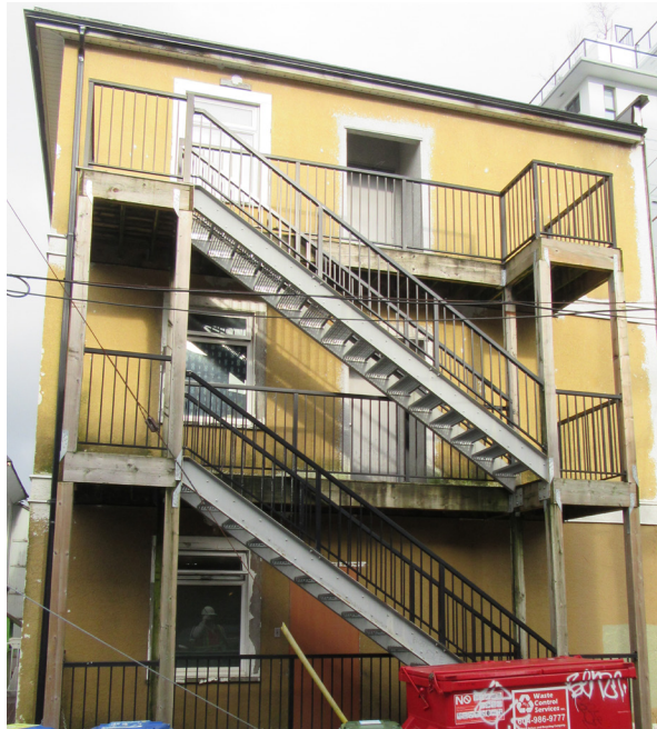
Door openings onto fire escape on rear elevation.
