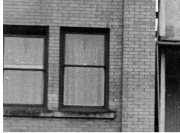
1958. Yates, A.L. 144 East 6 th Avenue [CVA Bu P508.15] showing original fenestration design (1-over-1 with sash horns).
