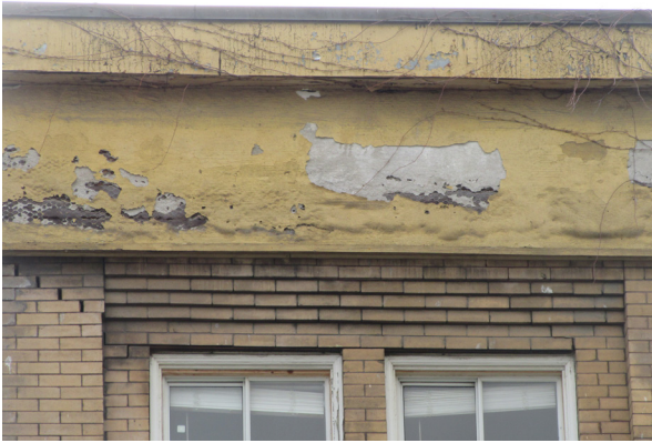
Brick corbel detailing above third floor windows.
