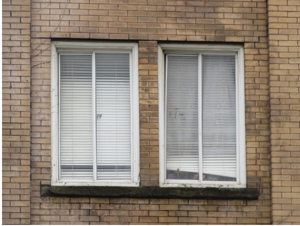
Original double assembly window openings on 3rd floor.
