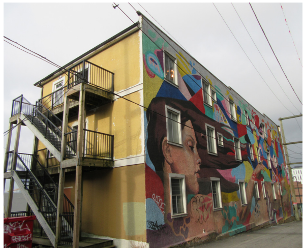
South-east corner of the Donnacona Block, standing at the side and rear laneways.
