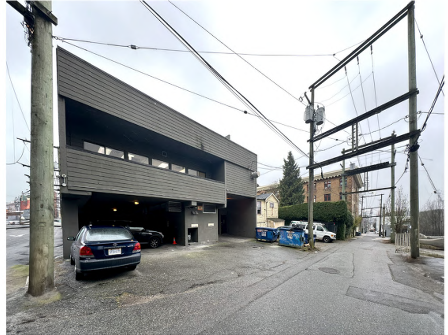
6 South Lane - View Looking towards south
