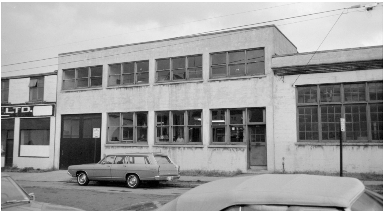
The 1942 extension building in 1973, location of Metalspray of BC Ltd. Source: Vancouver Archives CVA 1095-08871
