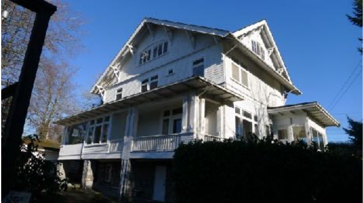
The house from the rear looking to the northeast showing the porch with its granite piers, the alterations with the expansion of a room into the porch cutting it in two. On the upper floors the two sleeping porches have been glassed in to provide additional living space.
