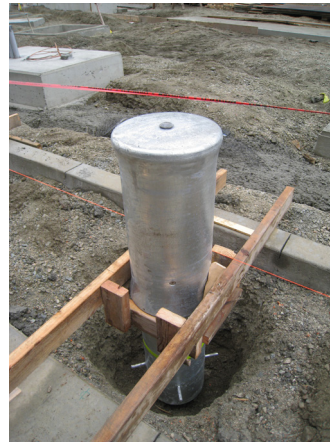
SEFC WATERFRONT BOLLARD. METAL CUSTOM GALVANIZED BOLLARD DETAIL AND INSTALLATION PICTURE.
