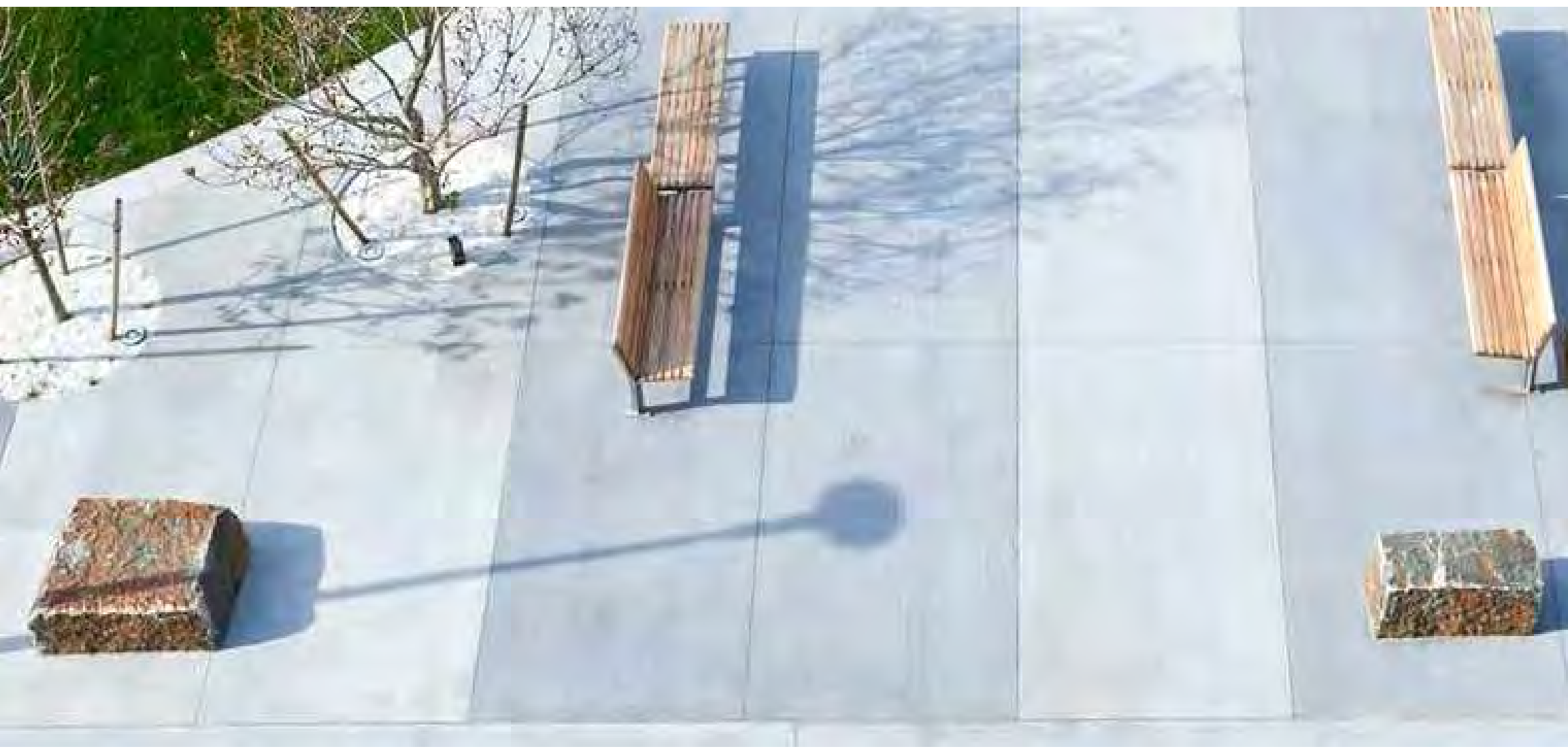
VEHICULAR CIP CONCRETE PAVING (PLAZA, HEALTHCARE BOULEVARD, SURFACE PARKING LOTS) PATTERN: 'WEAVE' INSPIRED
