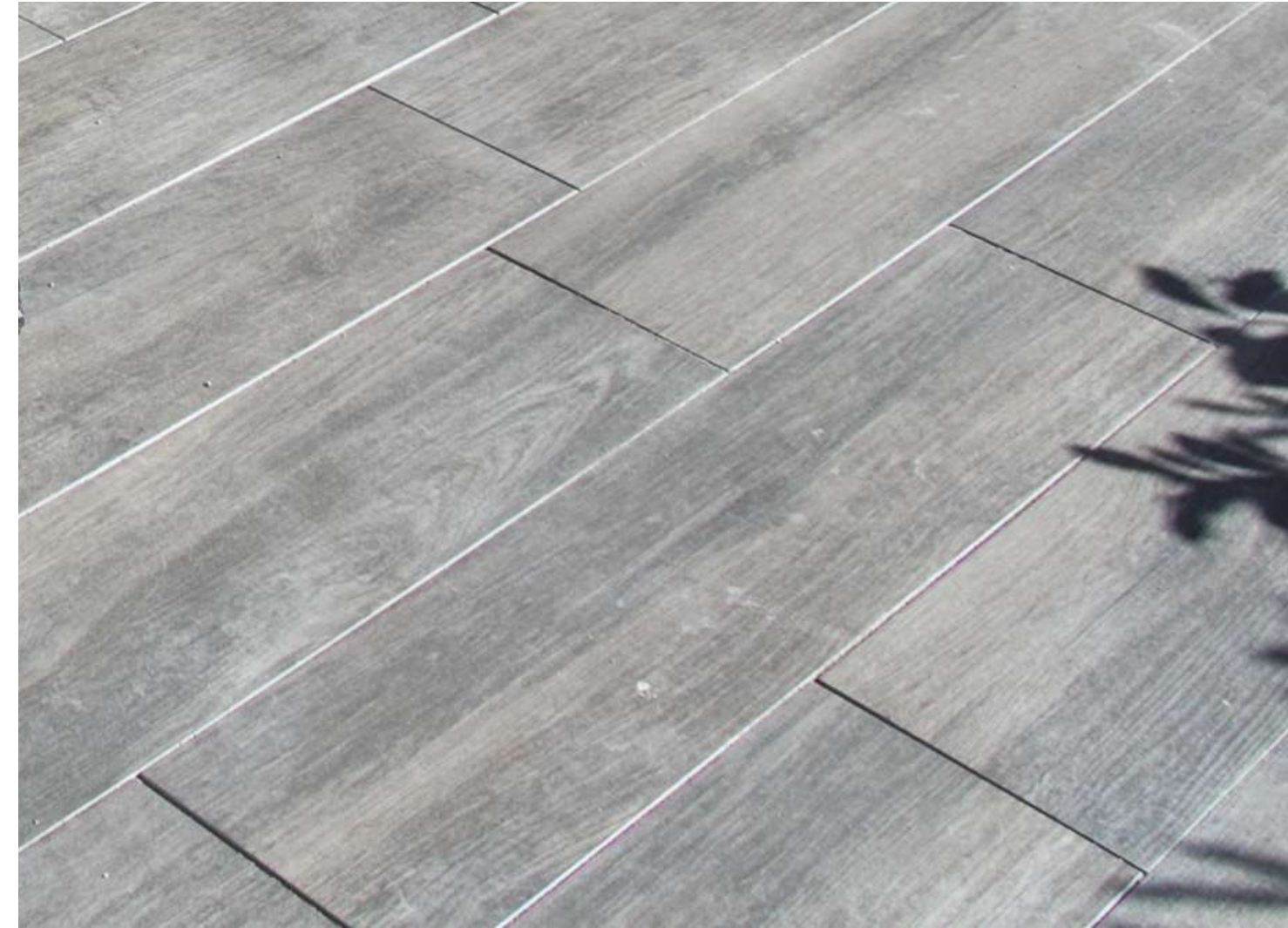
MODULAR PAVER SLABS PATTERN: LINEAR
