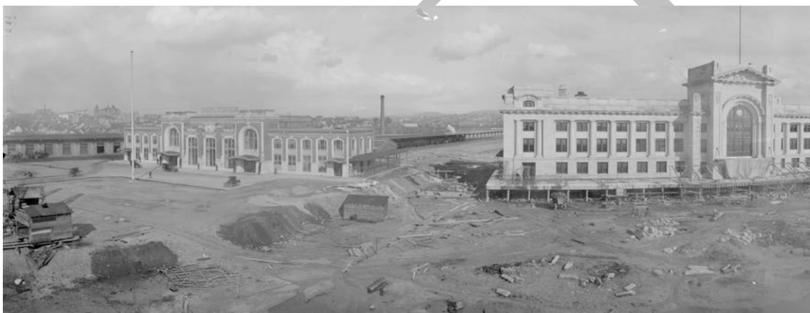
Figure 02. Union Station and freight depot (left) and Pacific Central Station (under construction, right) circa 1918.
