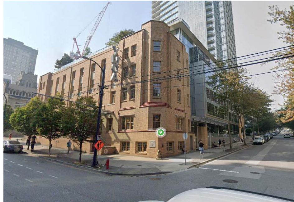
F. Burrard Street and Barclay Street frontages of the Robert Lee YMCA at 955 Burrard St.
