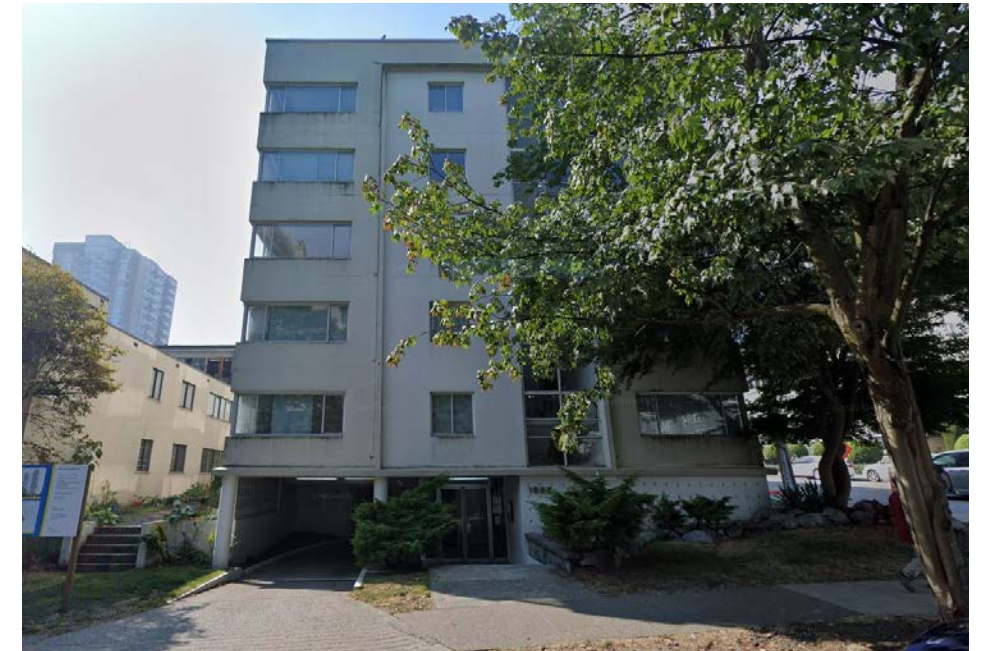
L. Barclay Street frontage of a 6-storey residential building.
