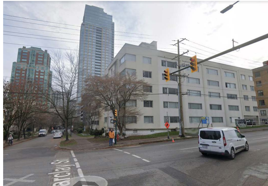
A. North and East frontages of 1080 Barclay Street, The Capri .
