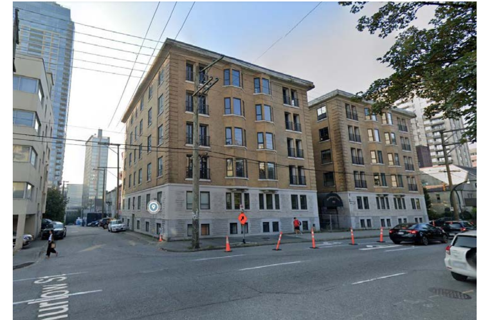
B. North elevation of Washington Court , a multi-family residential building at 998 Thurlow Street.
