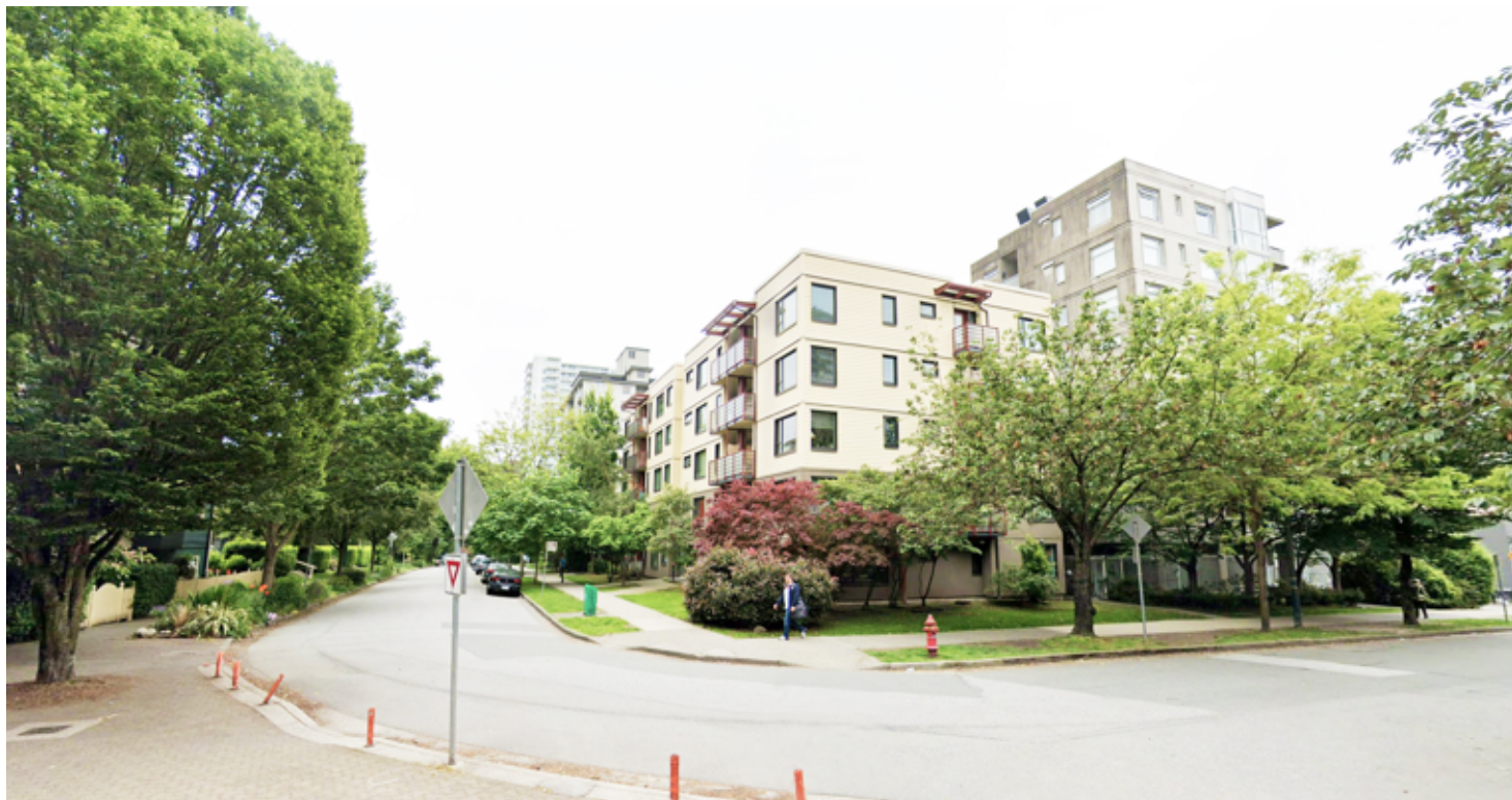
BUTE ST AND PENDRELL ST LOOKING SOUTHEAST
