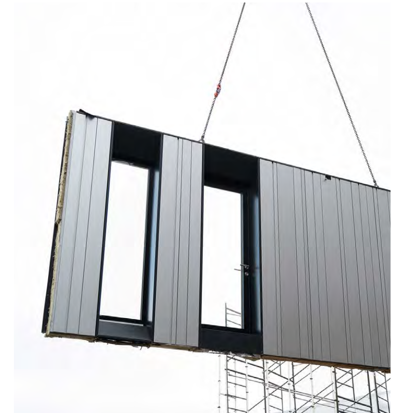
Performance Mock-up wall panel lifted into place
