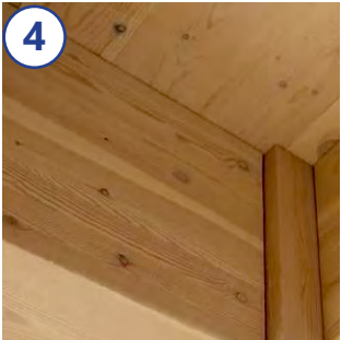
Glulam & CLT Glulam beams at ground floor canopy and CLT undersides exposed at rear balconies.
