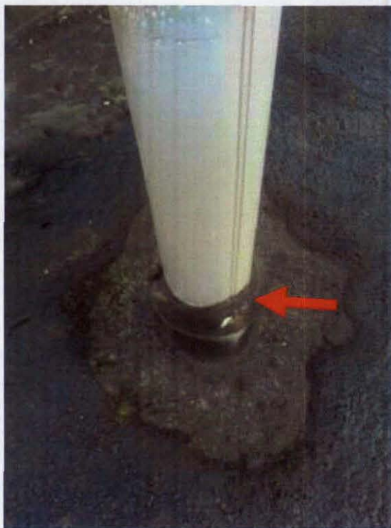
Photo # 1 – Asbestos-containing vent flashing mastic
