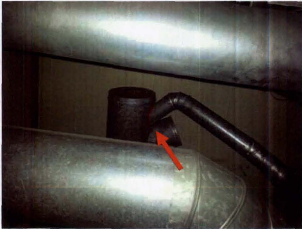
Photo # 7 – Assumed asbestos-containing red duct mastic
