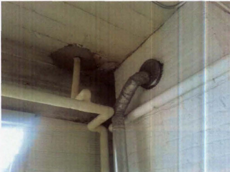
Photo # 6 – Asbestos-containing paring cement on pipe elbows within Suite 200.
