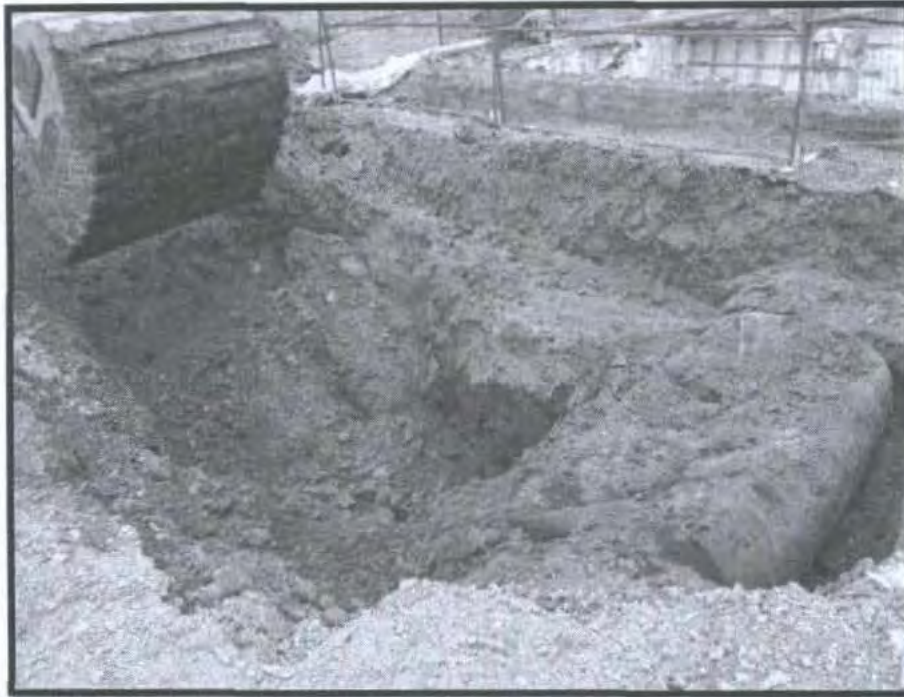
Photo 1 – Looking west. Uncovering of the former heating oil UST prior to tank decommissioning.
