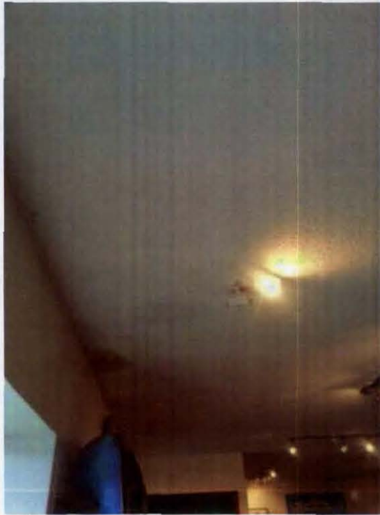
Photo # 5 – Asbestos-containing ceiling texture finish in Suite 301
