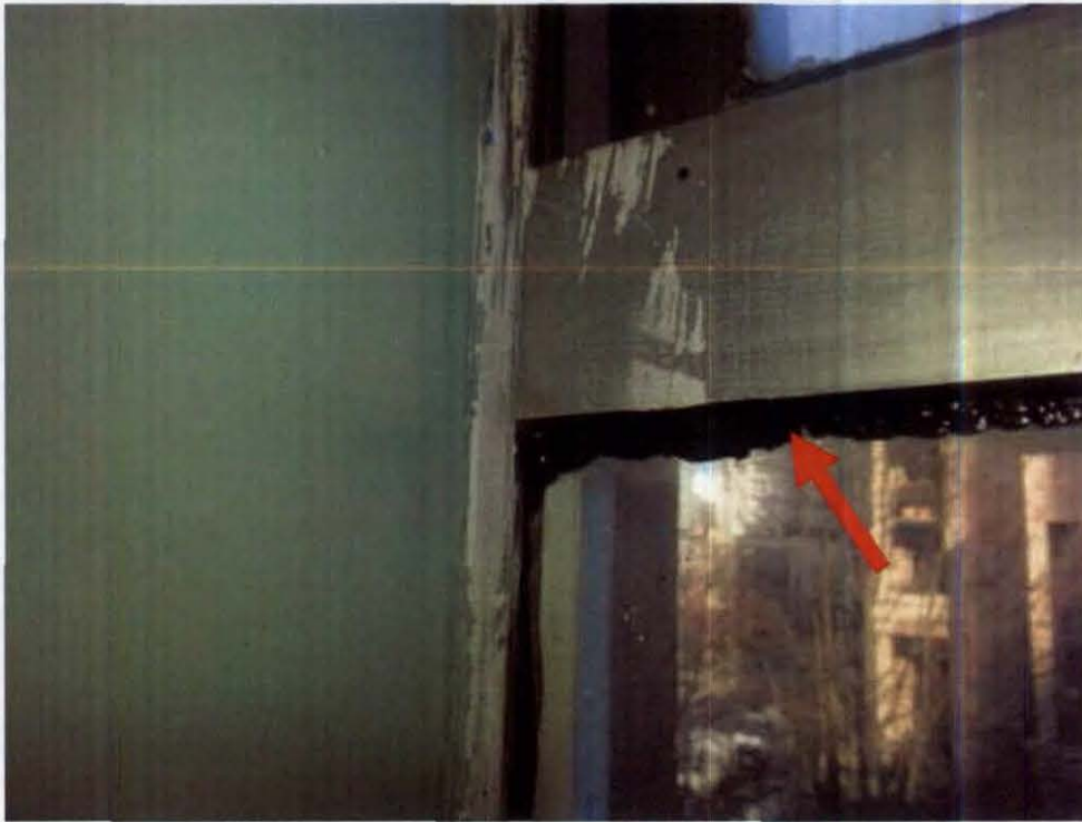
Photo # 3 – Asbestos-containing window glazing mastic
