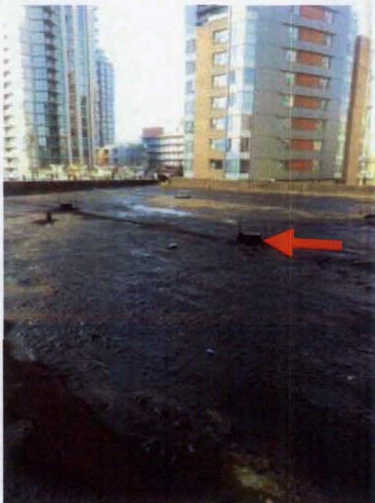
Photo # 2 – Asbestos-containing mastic on stumps
