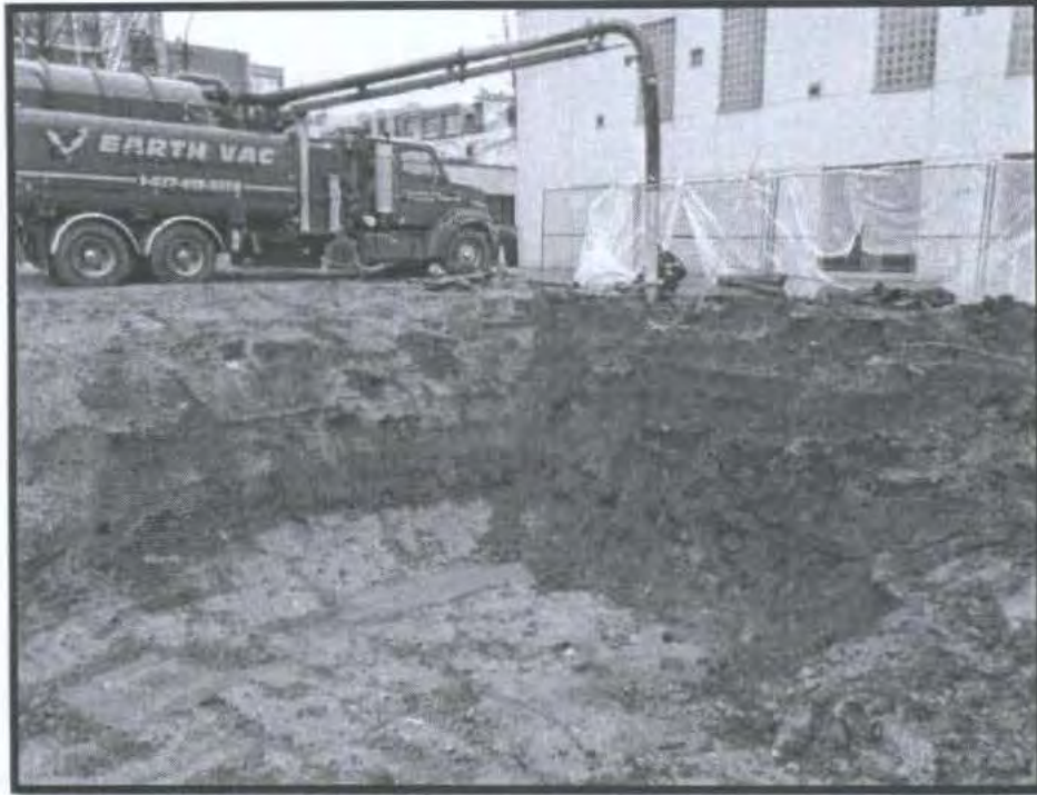
Photo 3 – Looking northeast. Shows the completed remedial excavation toward the lane and Drake Street Sidewalks. Residual soil at Site boundary to be removed during excavation trimming. Collection of closure samples shown via hydro-vacuum truck along Site boundary.
