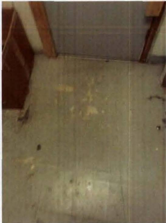
Photo # 4 – Asbestos-containing vinyl floor tiles present in areas on the 3 rd Floor
