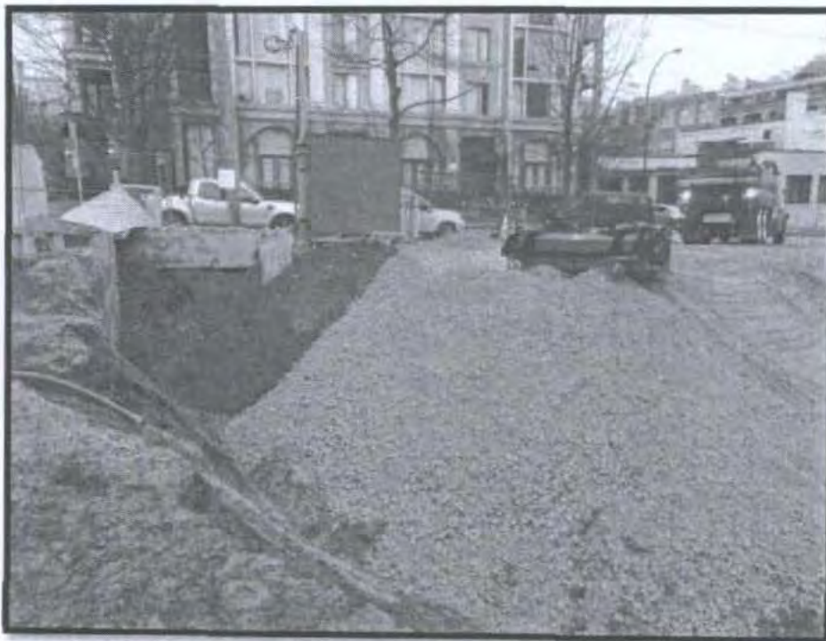
Photo 2 – Looking north. Shows the remedial excavation in the vicinity of the former UST. Backfill sand/gravel has been placed to support the adjacent Drake Street sidewalk.
