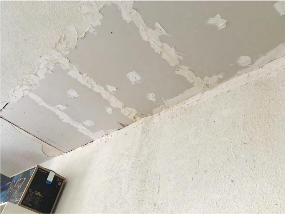
A photograph showing significant water damage to a ceiling and wall. Large sections of white drywall are missing, exposing a dark, brownish-grey substrate. The remaining drywall is peeling and stained. In the bottom left corner, a blue and black box is partially visible. | <p>s.22(1) Walls/ceiling - water damaged walls and ceiling.</p> <p>Violation #10</p> |
