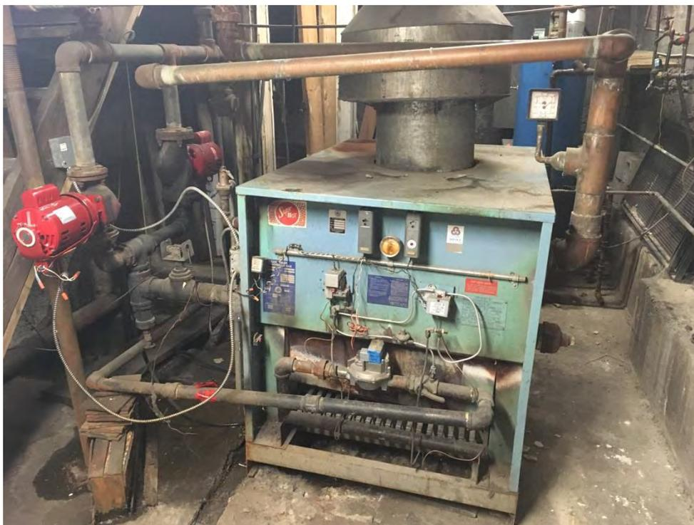
Furnace and associated mechanical systems in the basement are warm and appear and sound operational.
