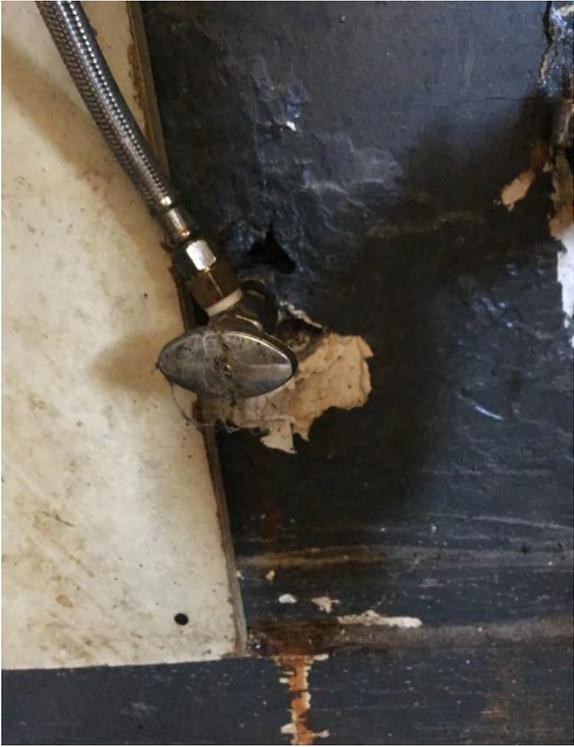
A close-up photograph showing a showerhead on the left, connected to a metal pipe. To the right, there is a hole in a dark, possibly waterproofed wall. The hole is irregular and appears to be a mouse hole. Some debris and a small amount of liquid are visible on the floor below the hole. | <p>s.22(1) Mouse hole in wall at water pipe.</p> <p>Violation #13</p> |
