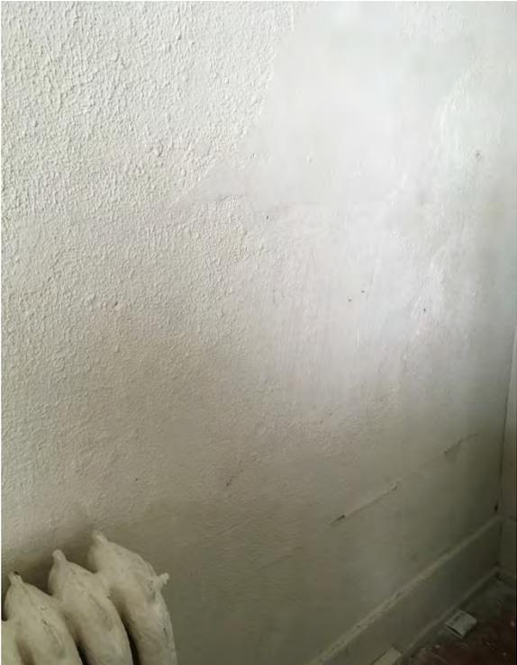
A photograph of a wall with unfinished drywall repair. The surface is uneven, with visible joints and areas of missing or poorly finished plaster. A white radiator is visible in the bottom left corner.                                                                      | <p>s.22(1) Walls - unfinished drywall repair.</p> <p>Violation #10</p>               |
