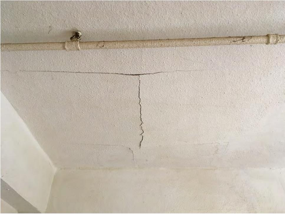
A photograph of a ceiling. A horizontal pipe runs across the middle. Below the pipe, there is a vertical crack in the white plaster. The ceiling shows signs of cracking and delamination.            | <p>s.22(1) Ceiling - cracked and delaminated plaster.</p> <p>Violation #8</p> |
