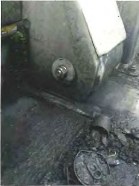
Westerly Roller bottoming out causing wear on frame and dragging ramp with float motion for excessive motion at top of ramp.
