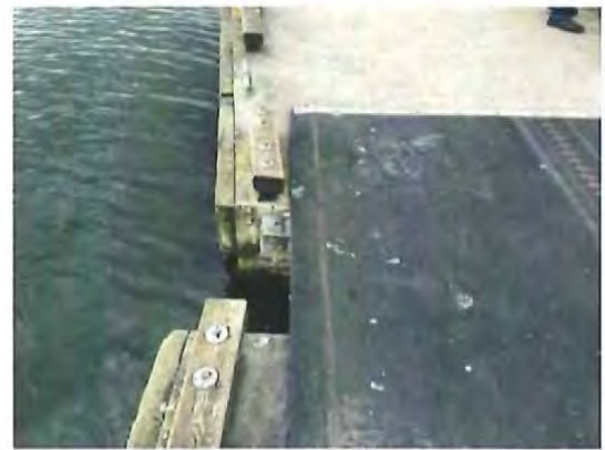
Figure 4-32: Excessive Gap Between Floats
