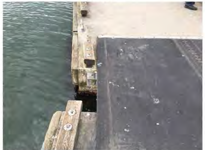
6 - Spalled Concrete
