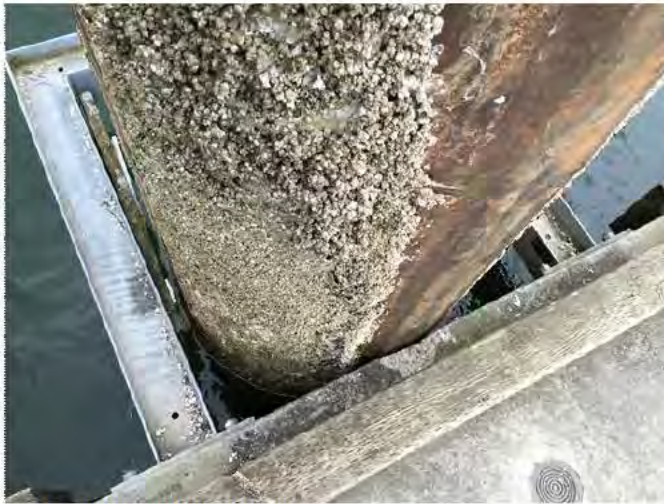
7 - Missing UHMW wear pad
