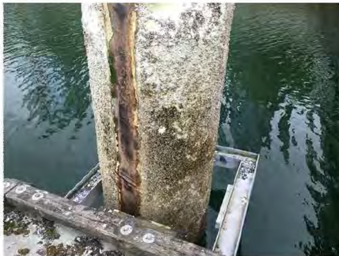
5 - Pile wear and corrosion
