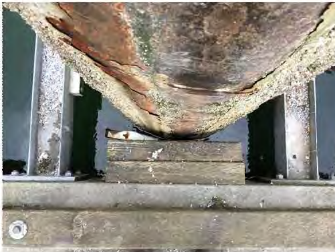
11 - Broken UHMW wear pad
