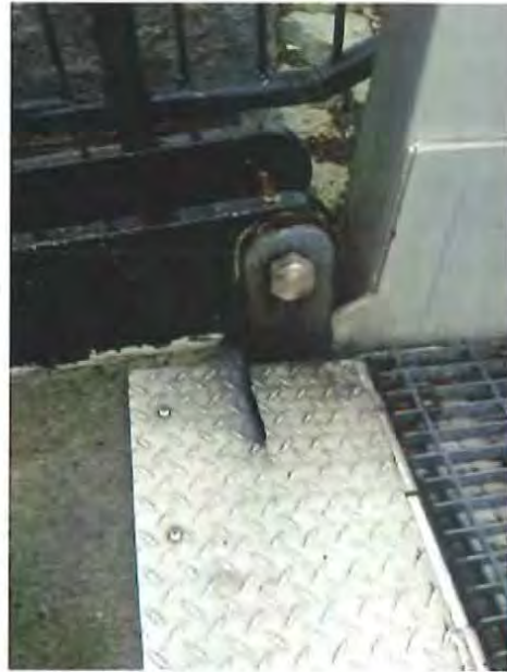
Westerly Link Plate and Transition Plate wearing excessively because roller is not rolling at seaward end of ramp.
