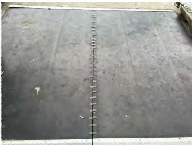
17 - 29 Deck Joints - Sheared Connection Links
