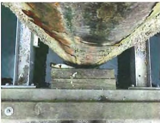
Figure 4-33: Deteriorated UHMW Sliders
