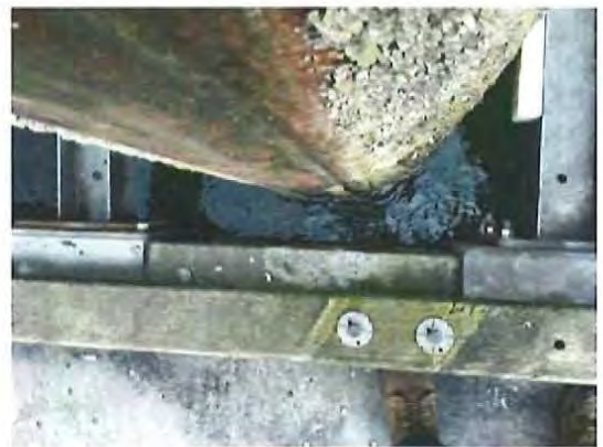
Figure 4-35: Missing UHMW Sliders
