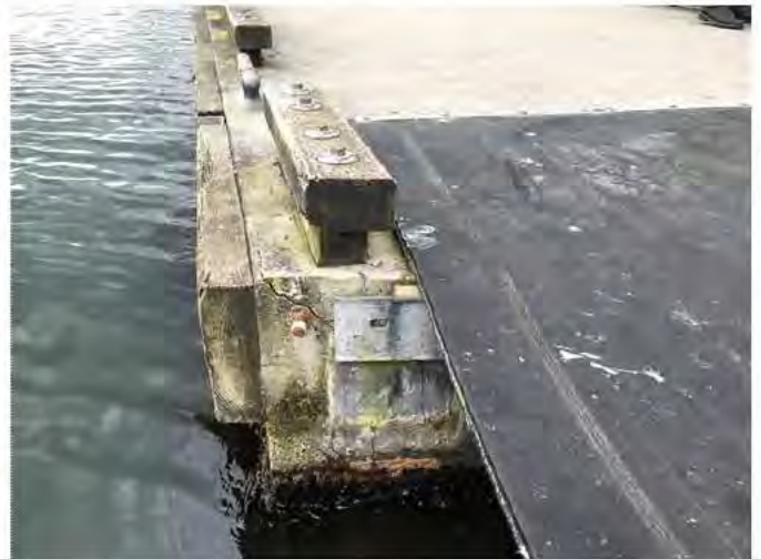
2 - Spalled Concrete
