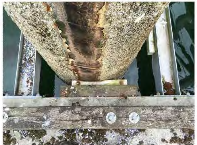
22 - Moss growth on concrete wearing surface
