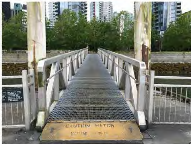
21 - Fungal growth on gangway guardrail
