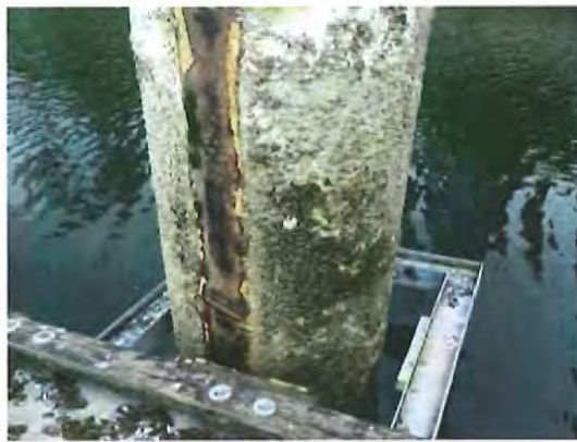
Figure 4-31: Abrasion to Mooring Piles
