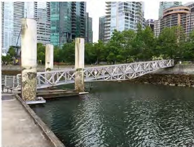
15 - Pile wear and corrosion
