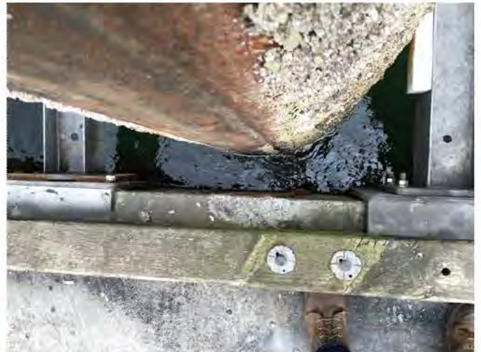
10 - Missing UHMW wear pad
