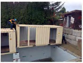
Mark and the professionals are believed to be the first in the Lower Mainland to build a RS-1 building using recycled steel construction. Mark designed the all electric, custom modular home in 2014. The building is prefabricated utilizing nine ISO shipping containers. The prototype build
