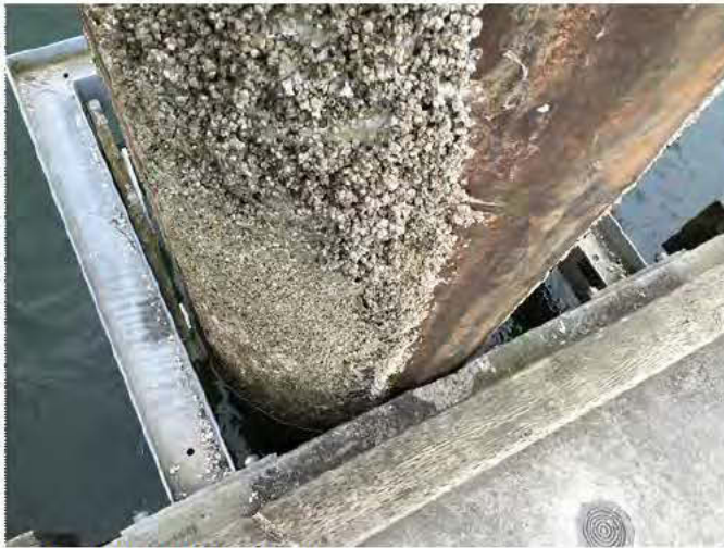
7 - Missing UHMW wear pad
