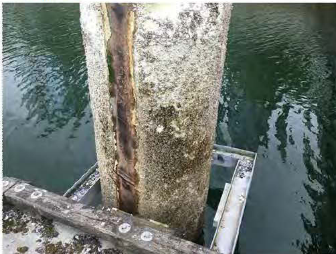
5 - Pile wear and corrosion
