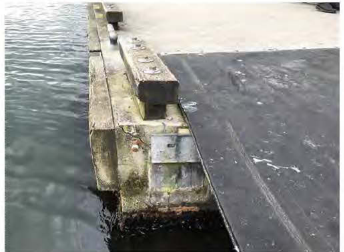
2 - Spalled Concrete
