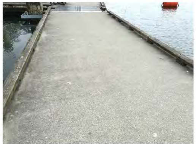
18 - Float 1 Wearing Surface, typical condition
