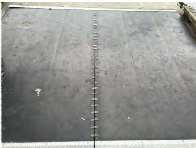
17 - 29 Deck Joints - Sheared Connection Links
