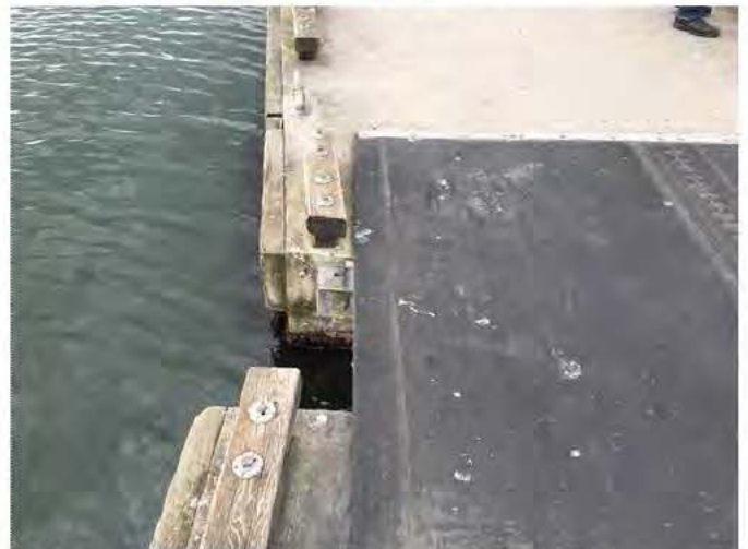
6 - Spalled Concrete
