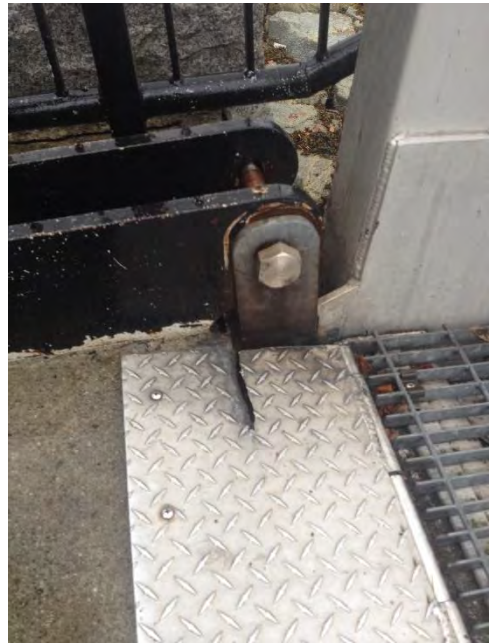
Westerly Link Plate and Transition Plate wearing excessively because roller is not rolling at seaward end of ramp.
