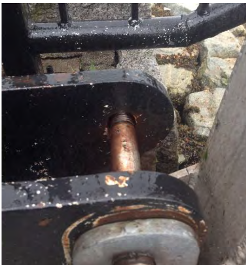
Westerly Roller bottoming out causing wear on frame and dragging ramp with float motion for excessive motion at top of ramp.
