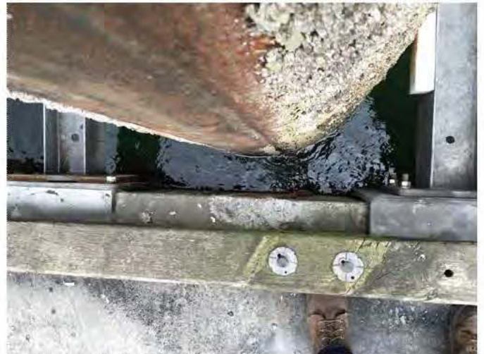
10 - Missing UHMW wear pad
