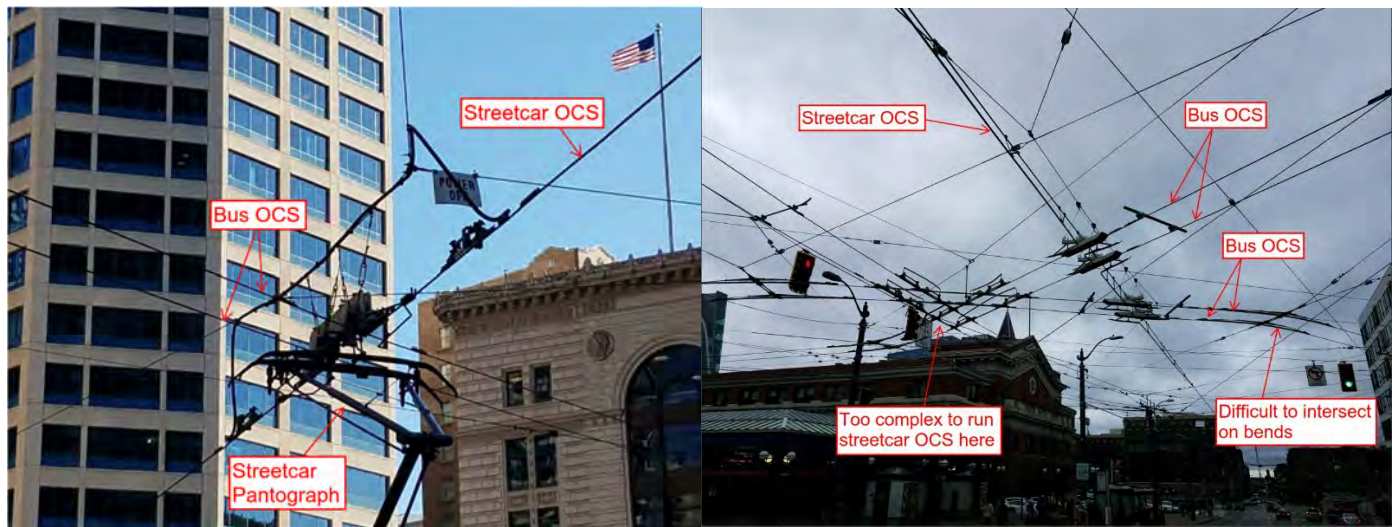
Figure 4-18 Seattle Streetcar and Trolley Bus OCS Intersections
