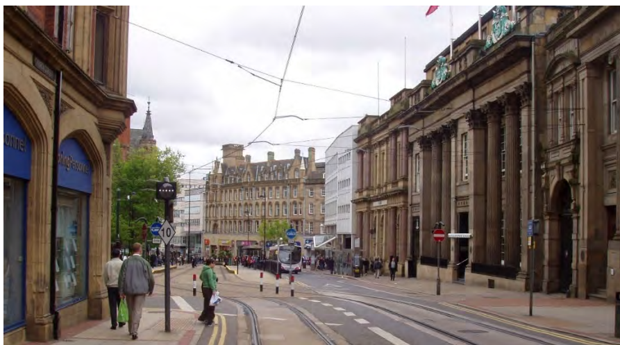
Figure 4-19 Simply Suspended OCS - Span Wires Affixed to Buildings, Sheffield, UK
