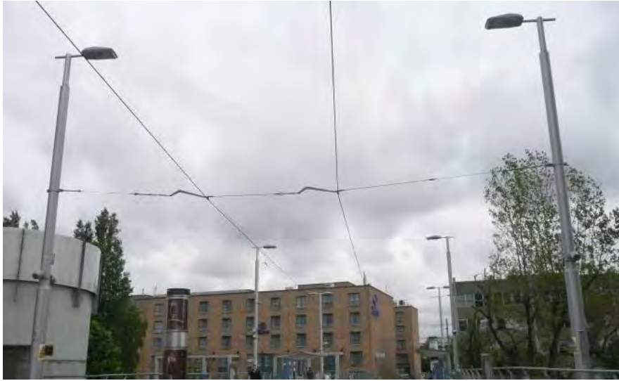
Figure 4-20 Simply Suspended OCS - Span Wires Affixed to Poles
