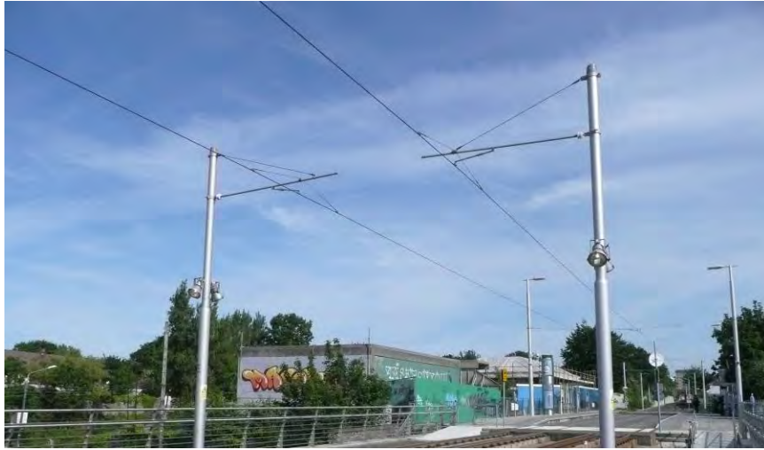
Figure 4-22 Bridle Suspended OCS - Affixed to Cantilever Poles
