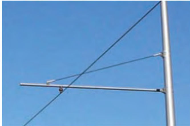
Figure 4-21 Simply Suspended OCS - Affixed to Cantilever Poles
