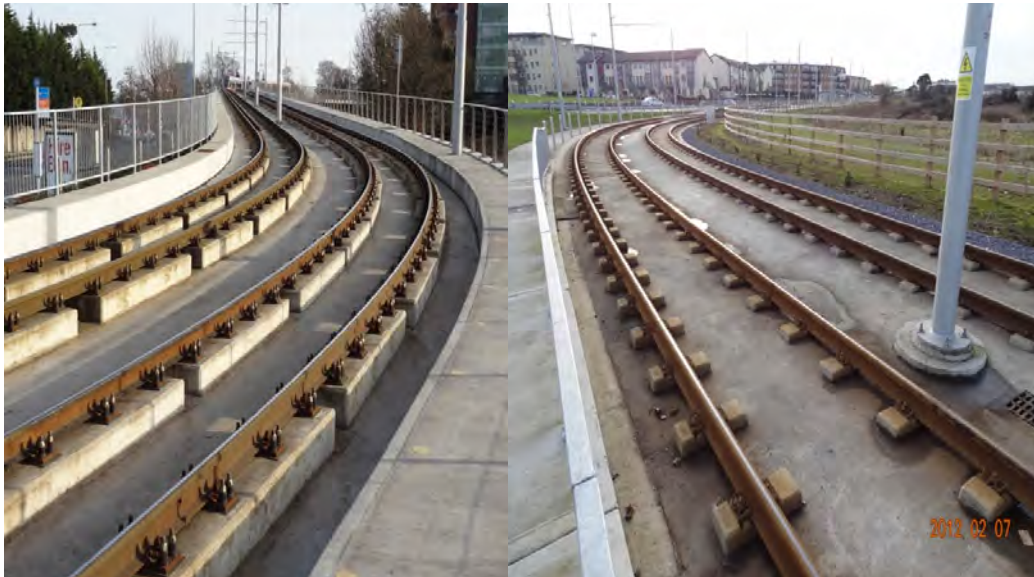
Figure 4-10 Direct Fixation Track from Dublin Luas
