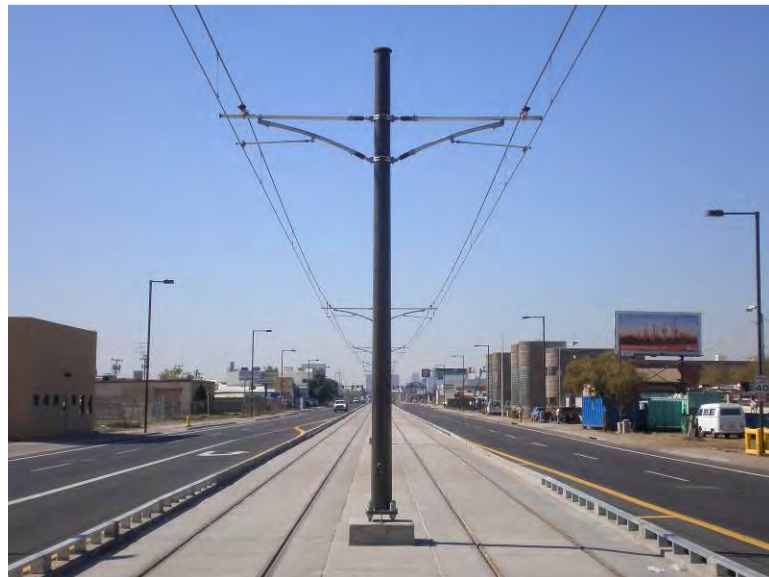
Figure 4-23 Simple Catenary OCS (Single Messenger Wire)
