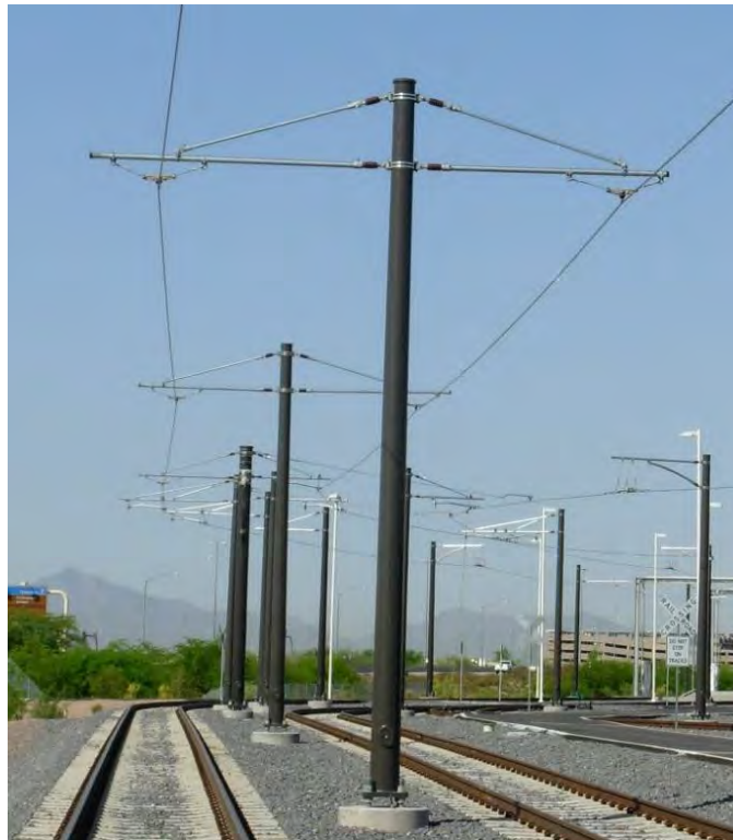
Figure 6-5 Dublin Luas with single wire OCS
