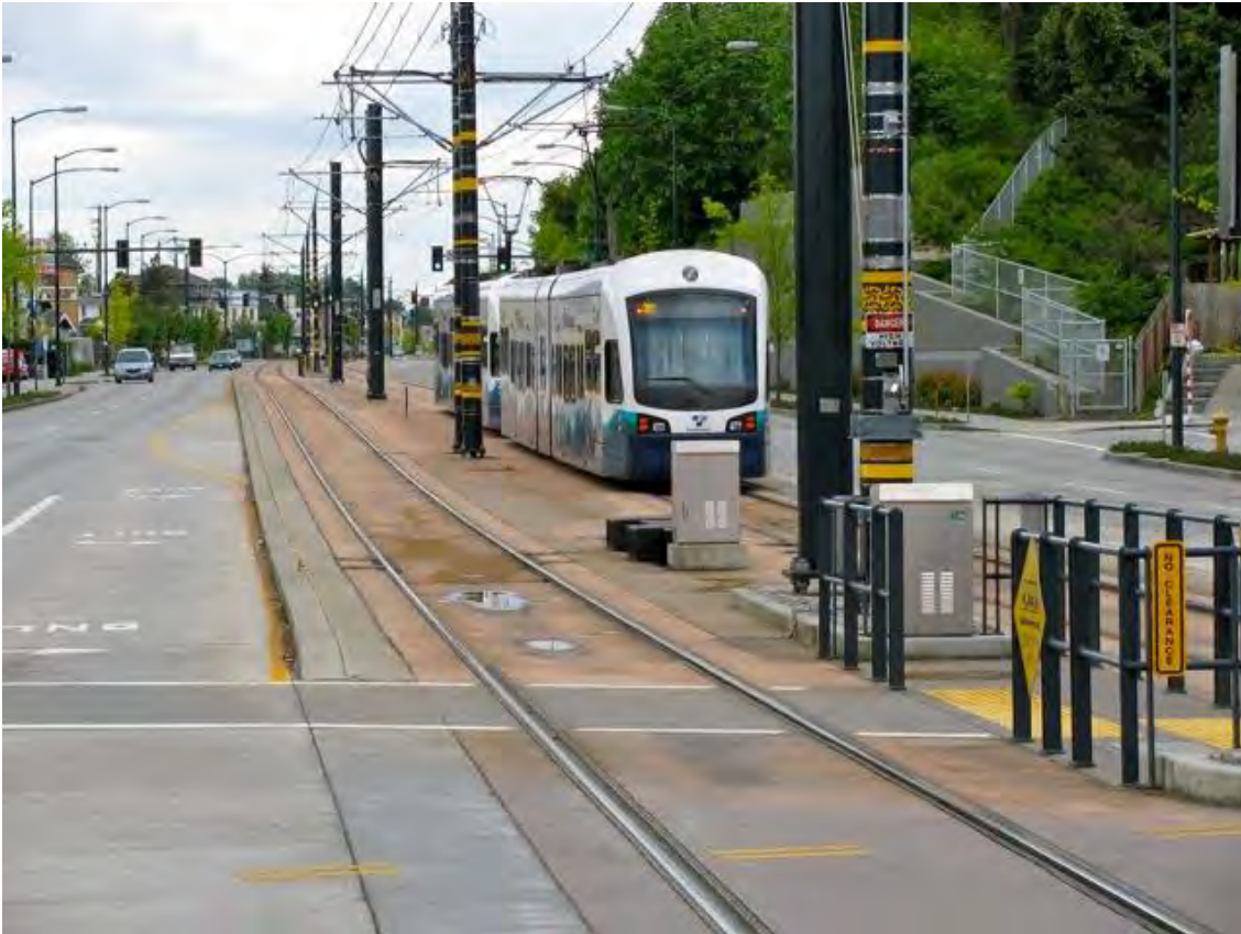
Figure 6-9 In-street Segregated Trackway, Seattle
