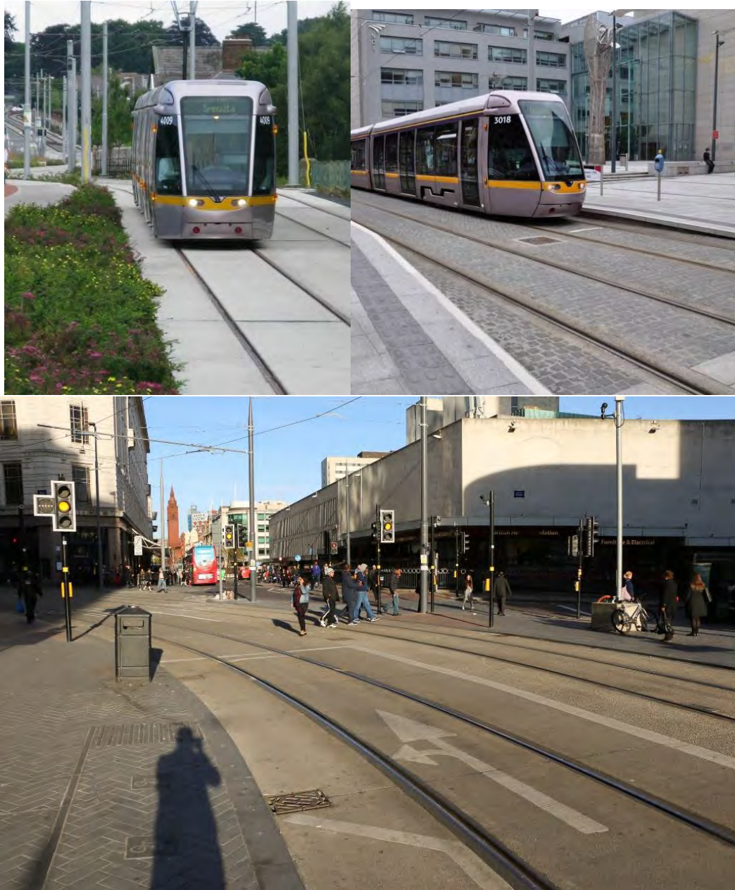
Figure 6-12 Embedded track from Dublin Luas and Midland Metro
