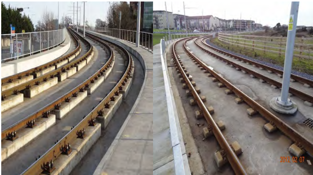
Figure 6-14 Direct Fixation track from Dublin Luas
