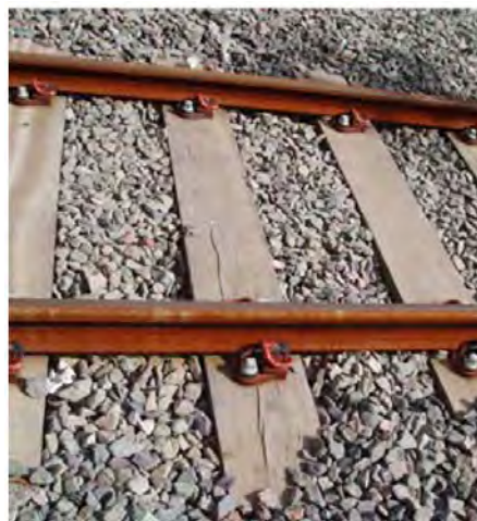
Figure 3: Ballasted track.
