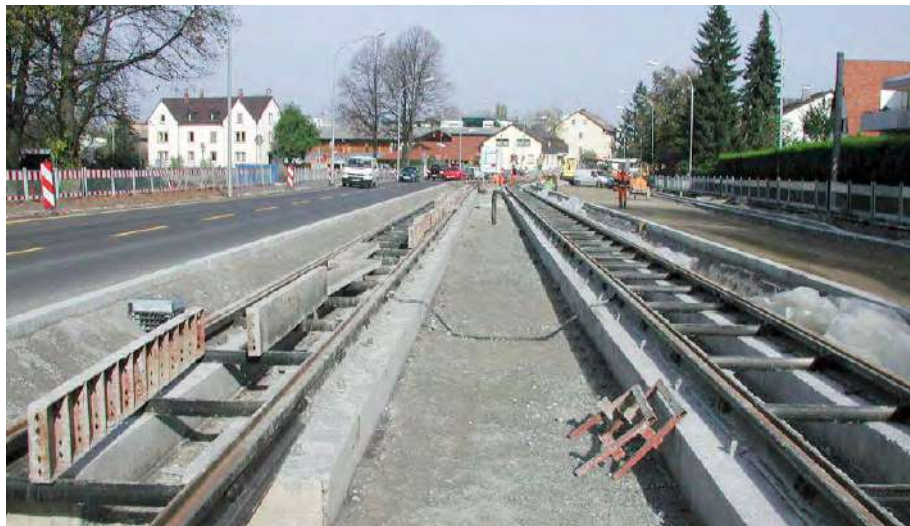
Figure 7: Construction of embedded grass track. Note additional depth between rails.
